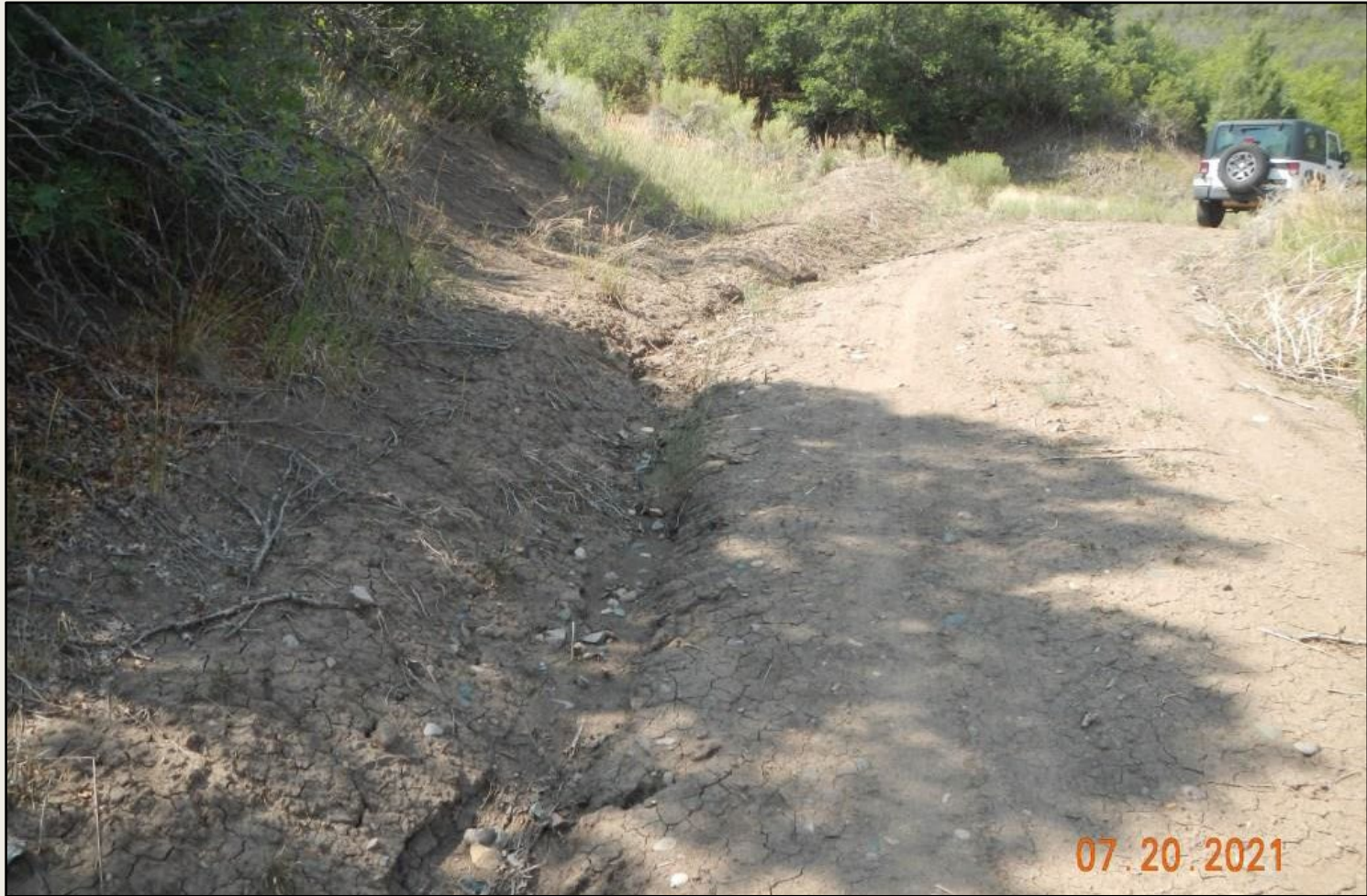
Photo 4. View of erosional channeling (approx. 12 inches wide and 4-6 inches deep) near the well pad entrance needing stabilization.
