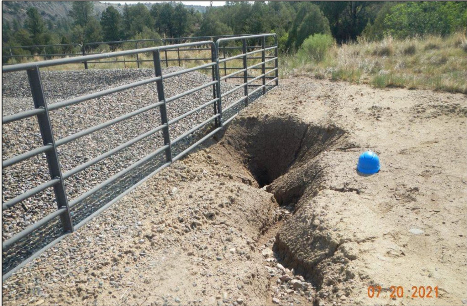
Photo 4. View of erosional tunnel in the northern project area approximately 3 feet wide (depth unknown).
