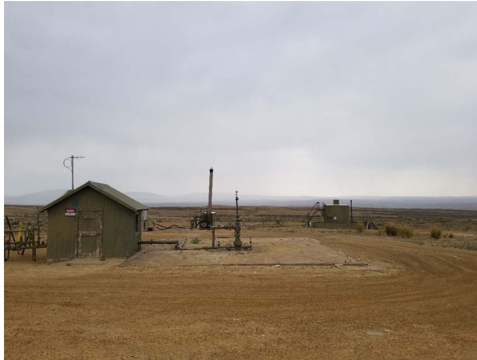
Photo 1. Overview of location taken facing north.
