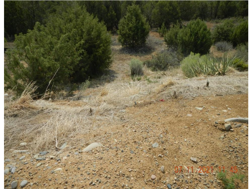
Wattles along eastern edge require maintenance.
