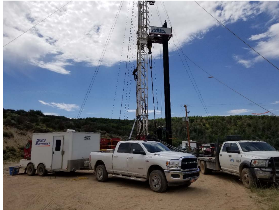
Photo 1. Overview of location taken facing south.
