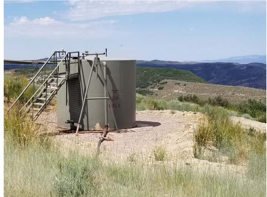
Photo 2. Tank labeled "emergency tank" no NFPA diamond.
