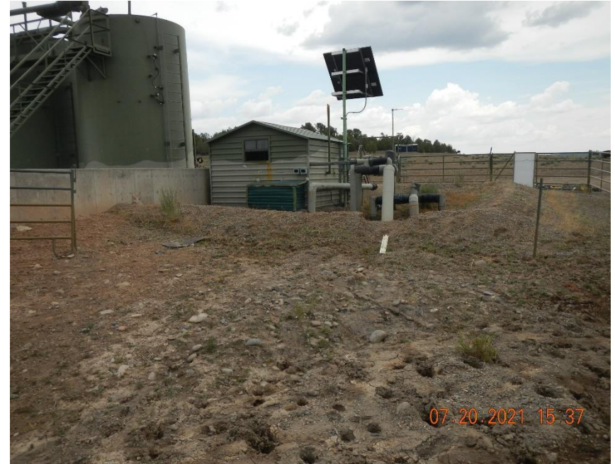
Down gradient view of secondary containment berm.
