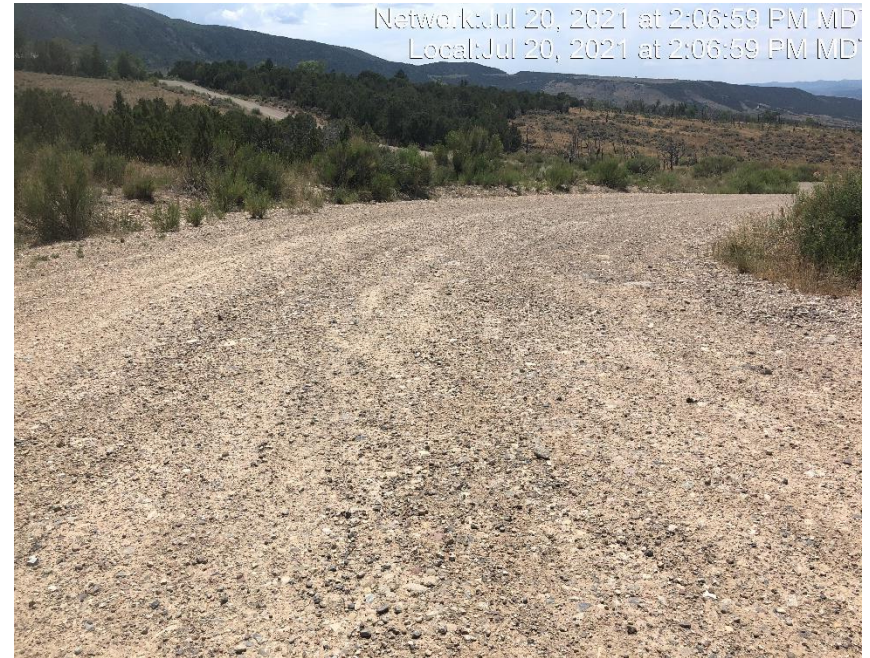
Photo #4511 no form of tracking BMP located at the entrance to location.
