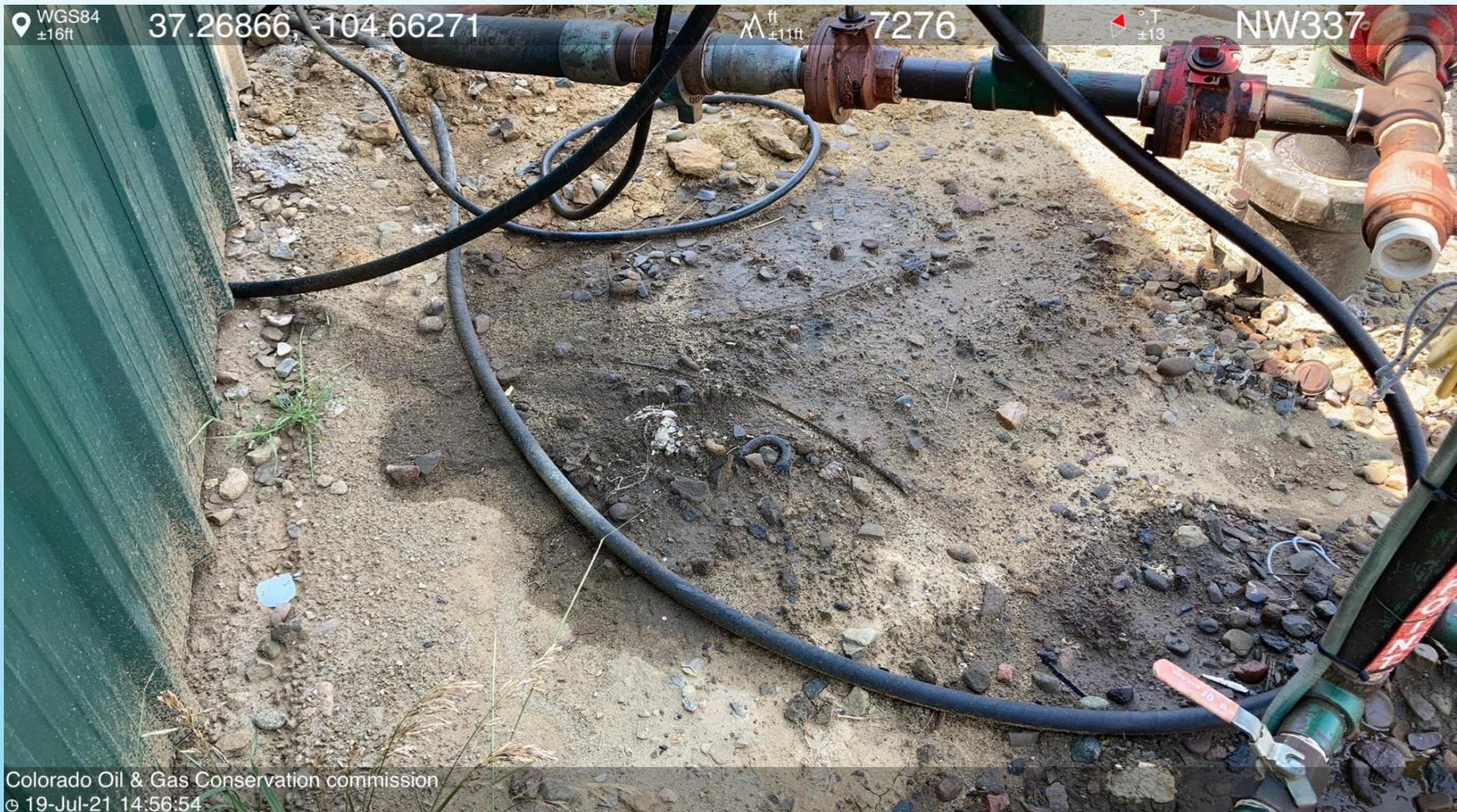
**PHOTO 4: ANOTHER IMAGE OF IMPACTED SOIL AROUND WELLHEAD.**
