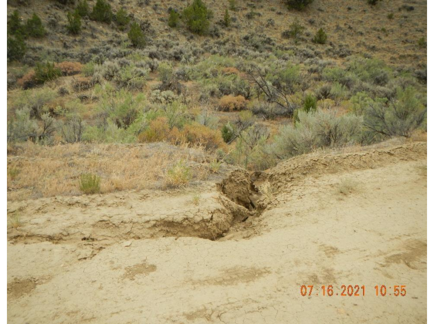
Storm water has washed out berm along access road. (40.08660 108.72430)
