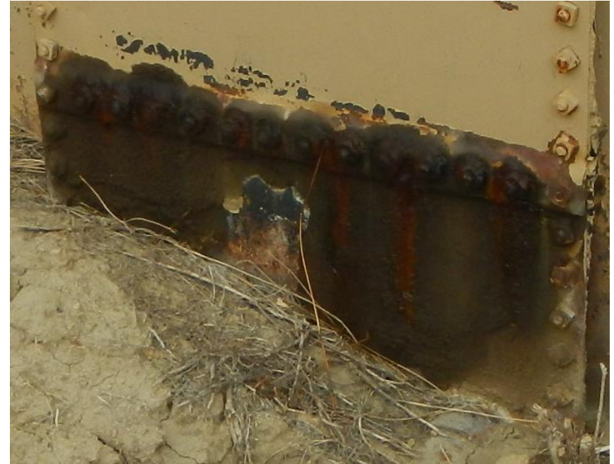
Oil seeping through bolts on man cover.
