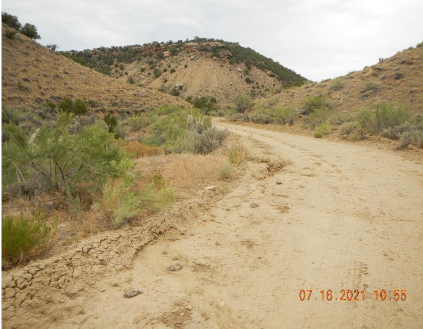
Sediment movement on roadside of access road.
