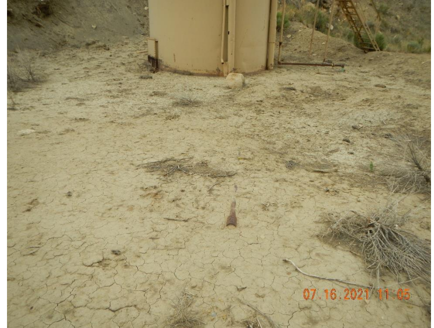
Unused open ended 2" tubing inside on tank berm.
