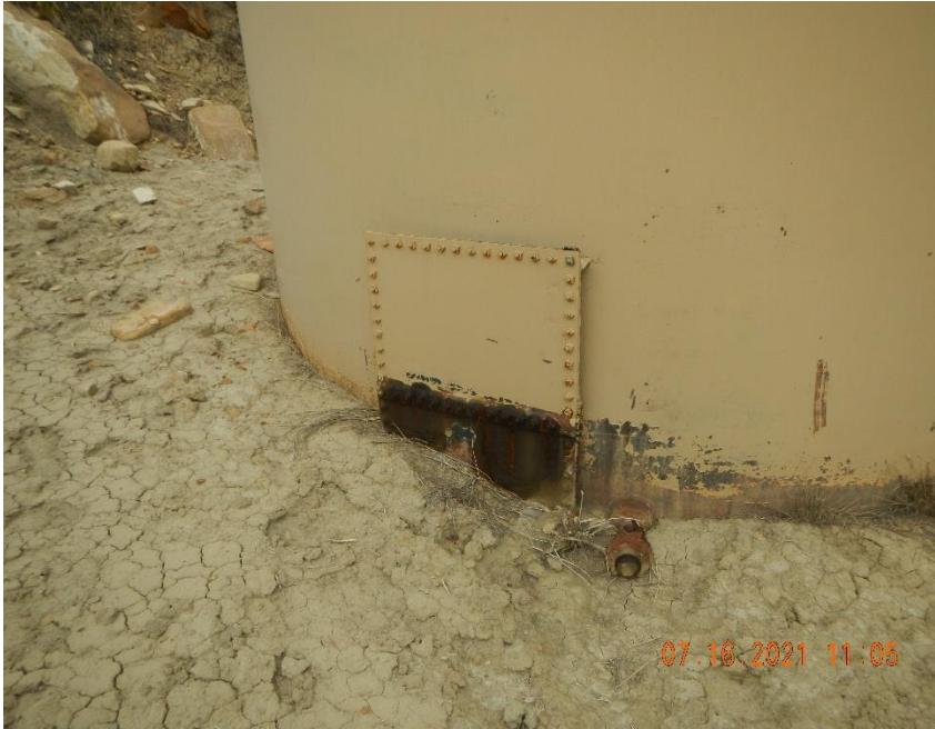
Sediment stacking against tank.
