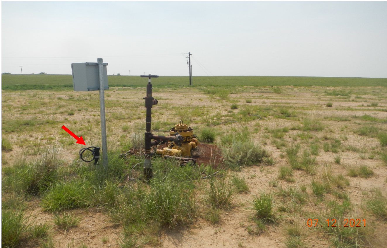
Photo 15. There is electrical wires extending out of the ground near the wellhead.
