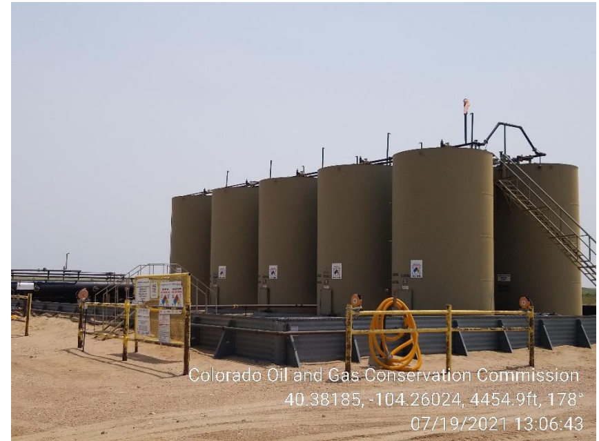
Photo 4 – Tank Battery
