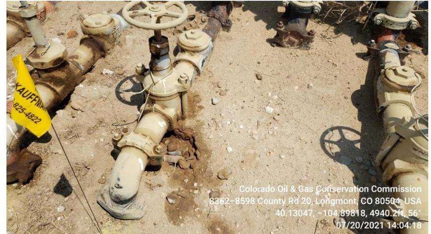
**Photo 17 Stained soil by the Flow line manifold**
