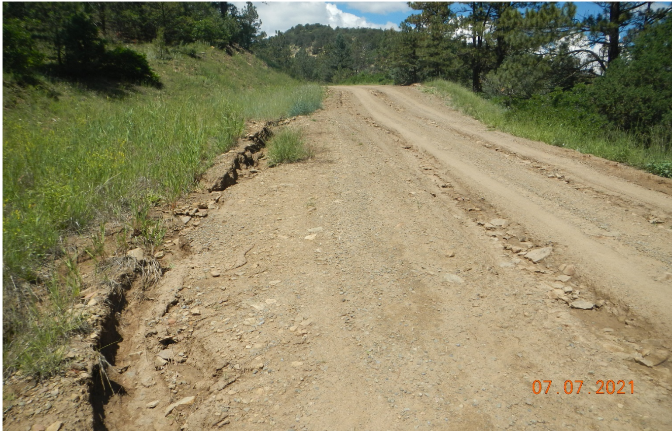
Photo 3. Storm water erosion is occurring down the side of the road. BMP's need to be installed to prevent erosion. Previous corrective action was not performed.
