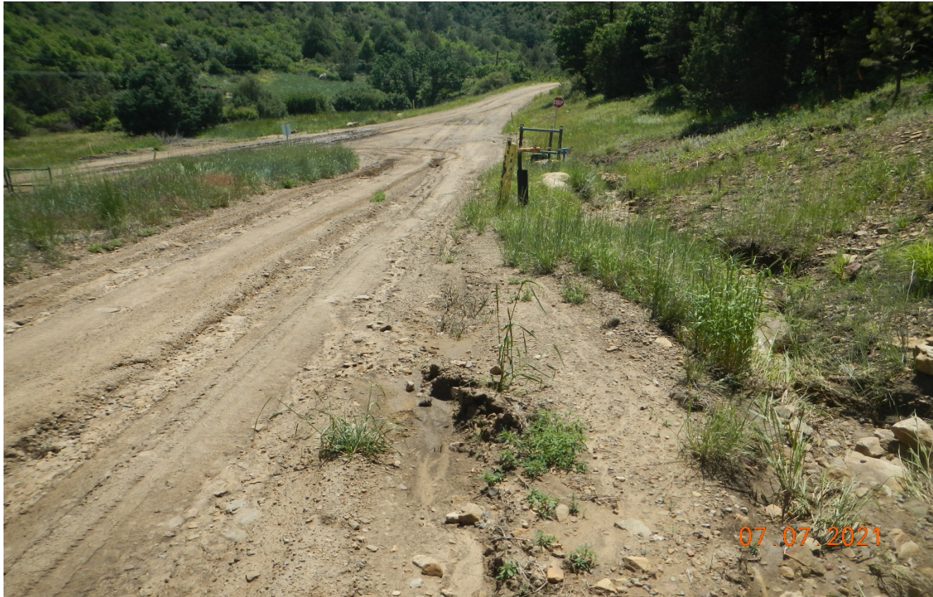
Photo 2. Facing back down the access road shows vehicle rutting and erosion. This issue has previously been documented and needs to be repaired and prevented.
