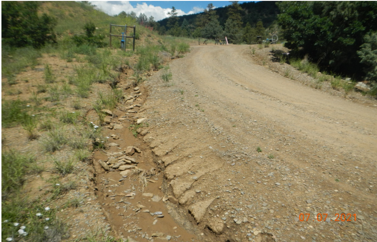
Photo 4. Facing along the access road toward the location. Storm water erosion is occurring down the side of the road. BMP's need to be installed to prevent erosion.
