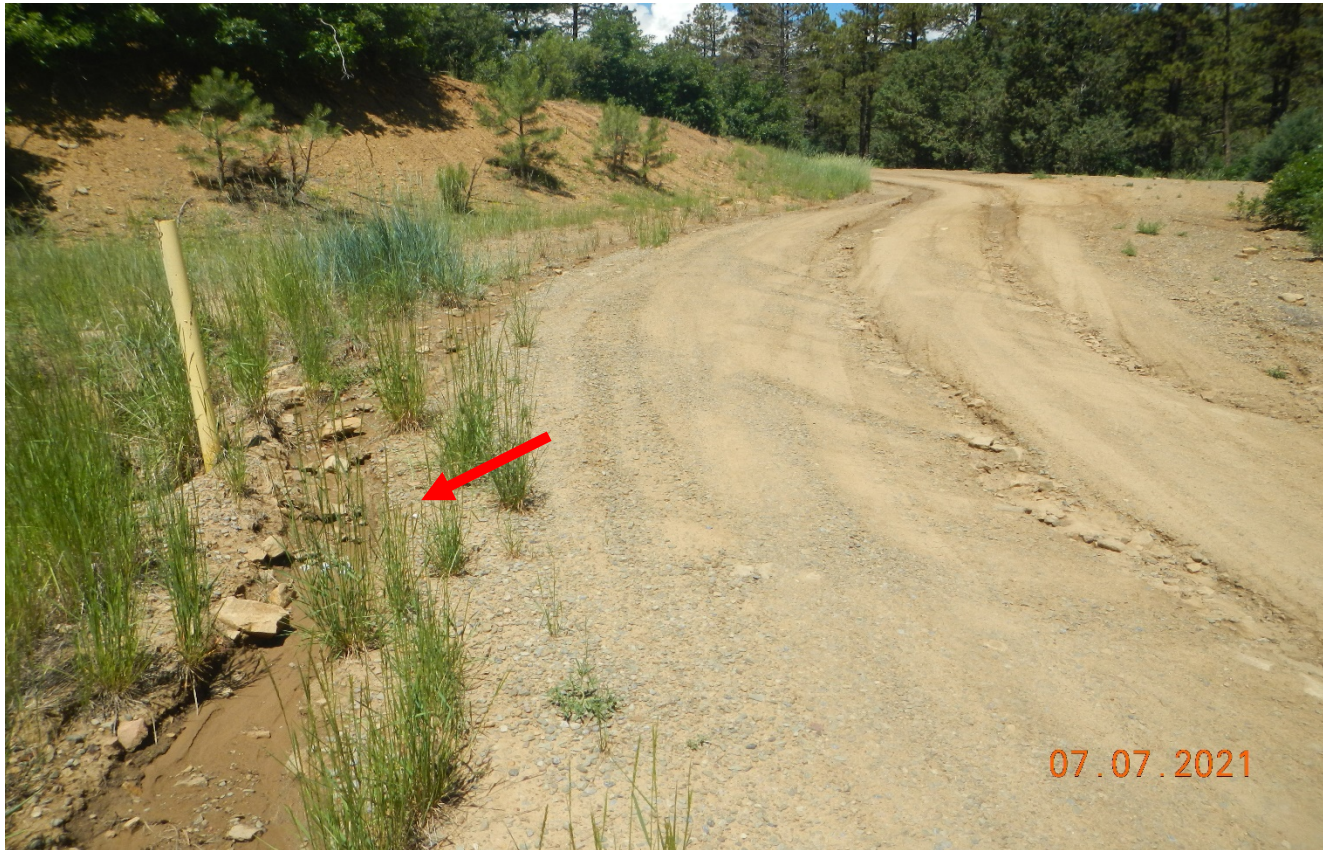
Photo 4. This is the same culvert shown in previous photo which stormwater not properly diverted to the culvert causing erosion.
