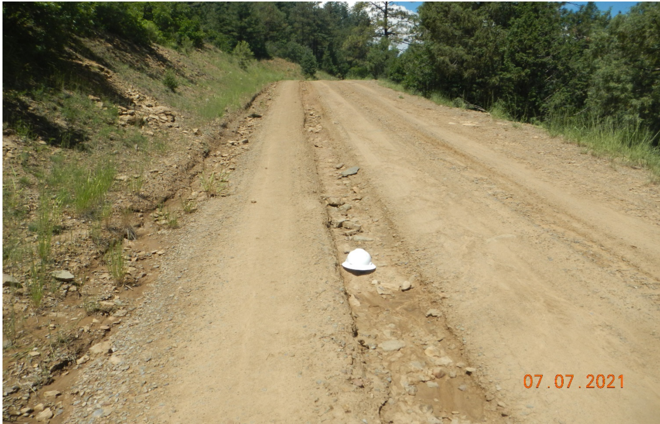
Photo 1. There is vehicle rutting and erosion along the road. The white hard hat is placed in the vehicle rut for scale.
