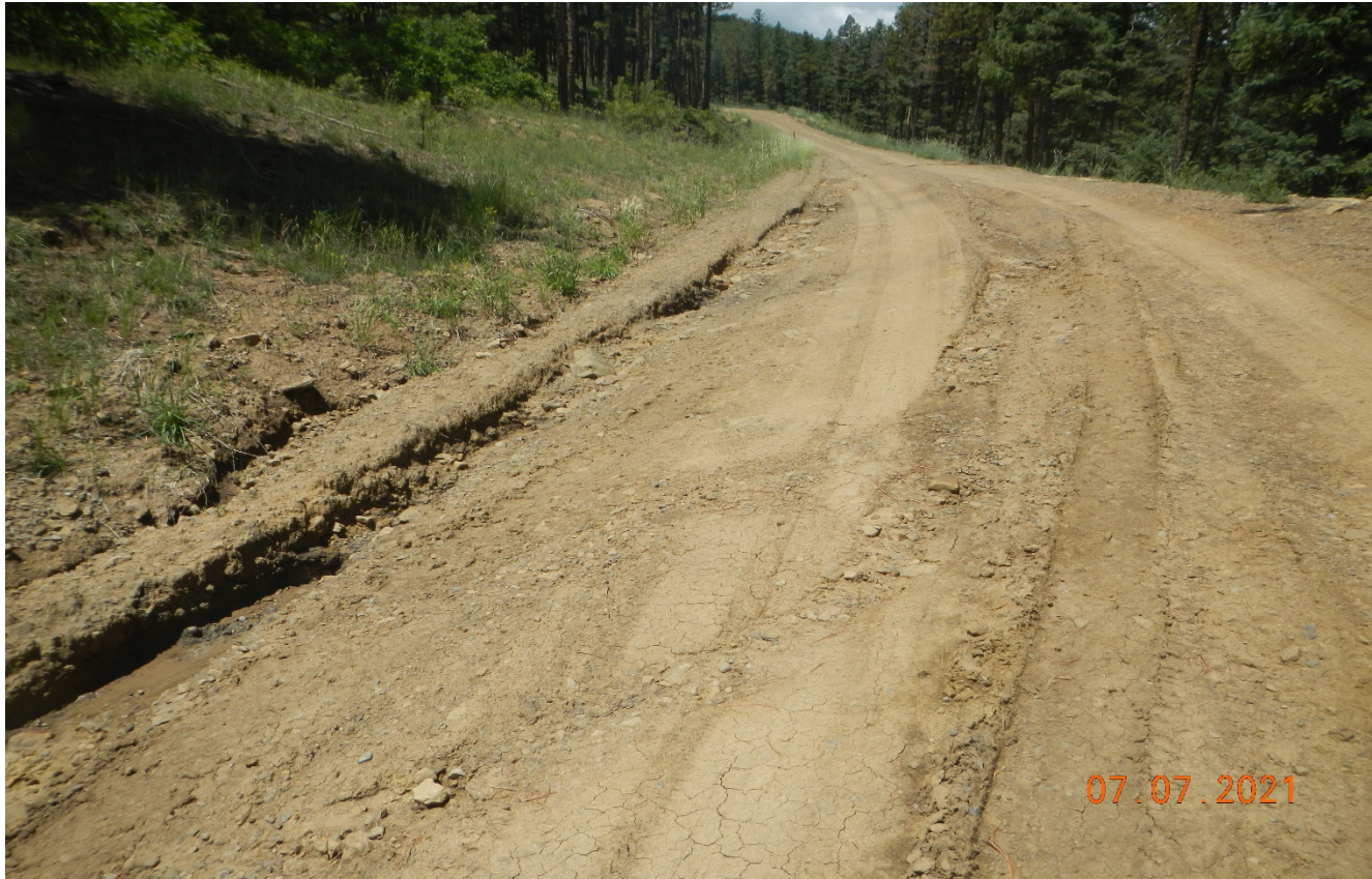
Photo 5. There is vehicle rutting occurring along the road which will only worsen if not repaired. The roads need to be maintained. Previous corrective action was not performed.
