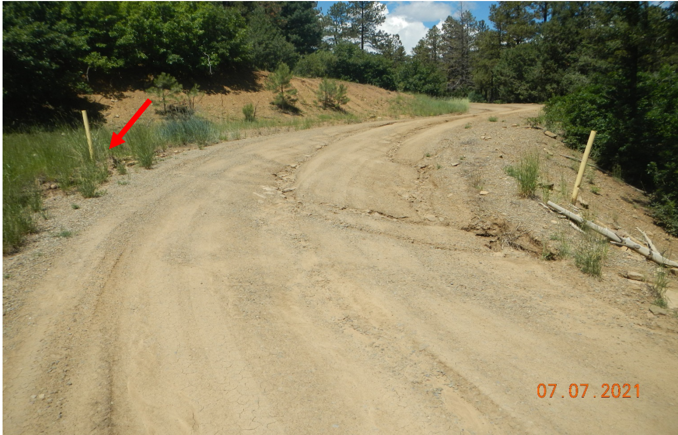
Photo 3. Stormwater is not being diverted toward the culvert (red arrow) and is flowing across the road causing erosion.
