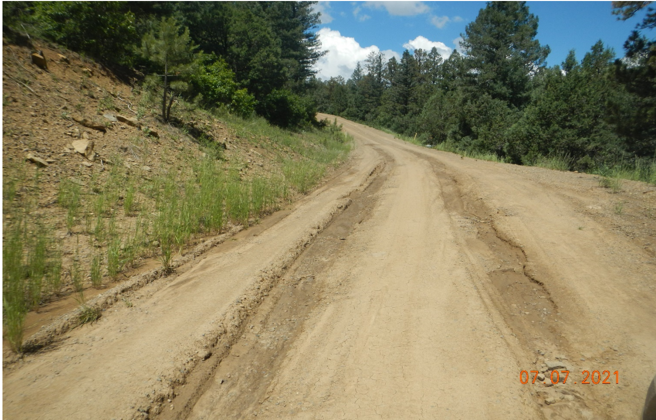
Photo 2. There is vehicle rutting and erosion along the road. Previous corrective action was not performed.
