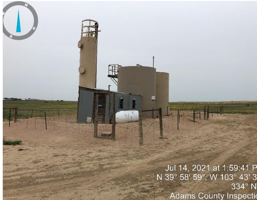
Photo #3 Separator & tanks.
