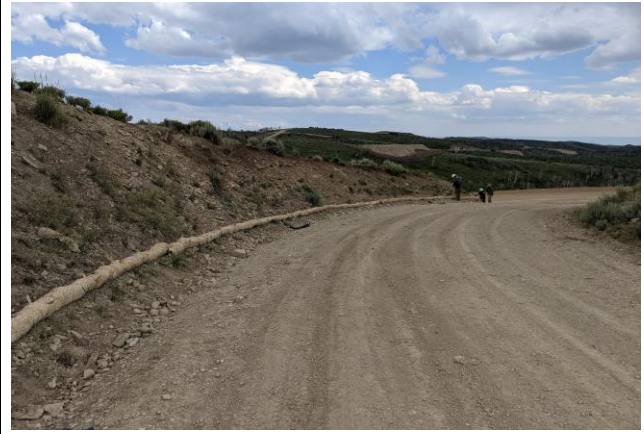
Installing Wattle on CC 603-23-32 Pad
