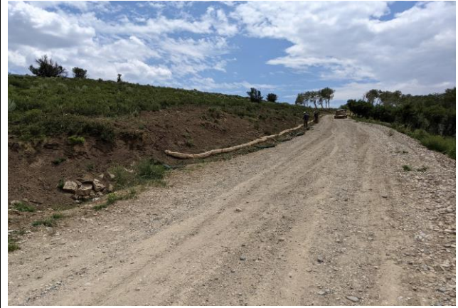
Installing Wattle Along the CC 697-03-07 Access Road
