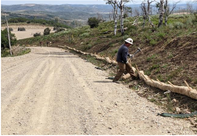
Installing Wattle Along the CC 697-03-07 Access Road
