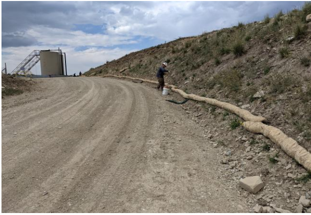
Installing Wattle on CC 603-23-32 Pad
