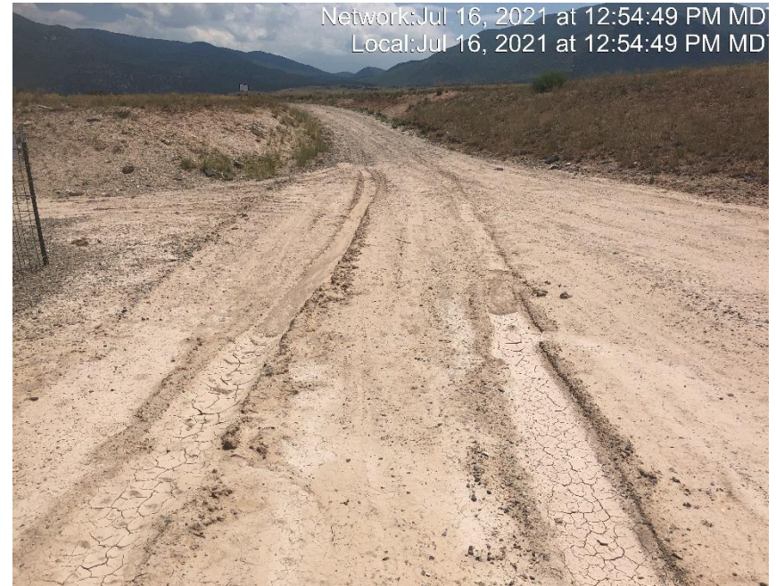
Photo #4475 No form of tracking BMP located at entrance to location.
