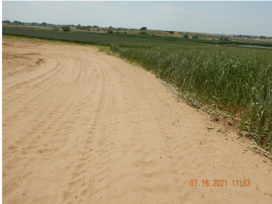
Photo 8. Photo taken from the northwestern location, facing West. Photo illustrates Operator has failed to install perimeter stormwater BMPs during construction activities.
