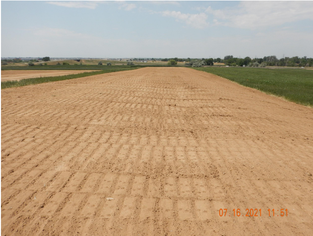
Photo 7. Photo taken from the northern location, facing West. Photo illustrates the topsoil stockpile which has been temporarily stabilized with equipment tracking.
