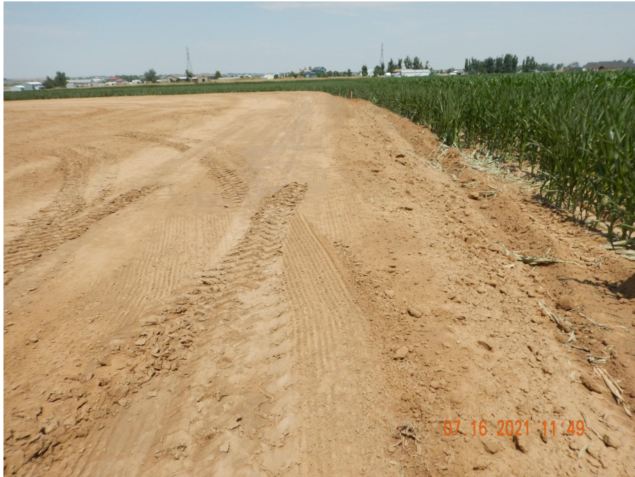
Photo 5. Photo taken from the northeastern location, facing North. Photo illustrates Operator has failed to install perimeter stormwater BMPs during construction activities.
