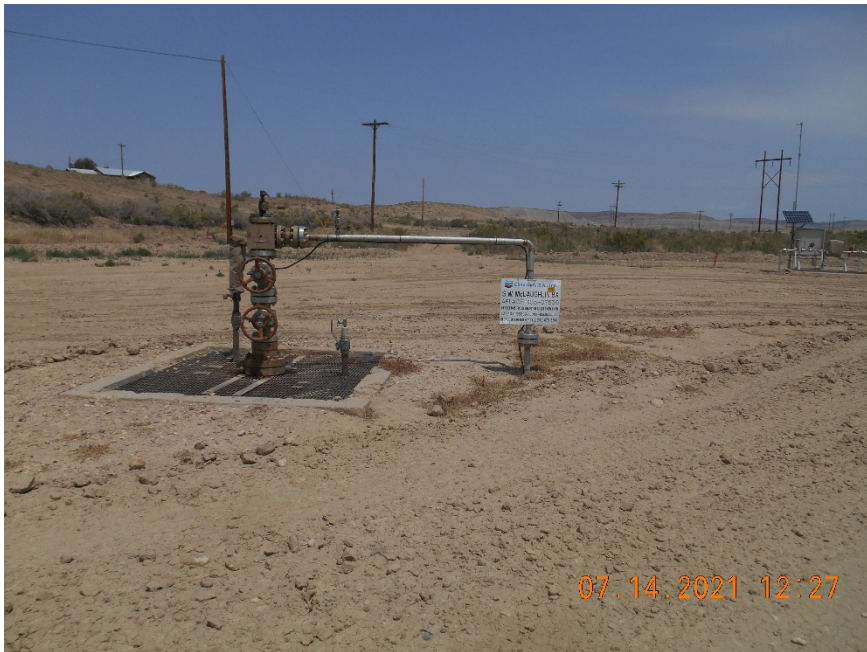
Injection wellhead.
