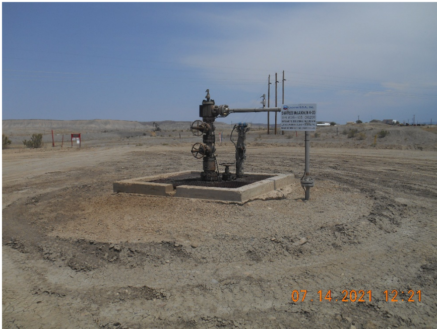
Injection wellhead
