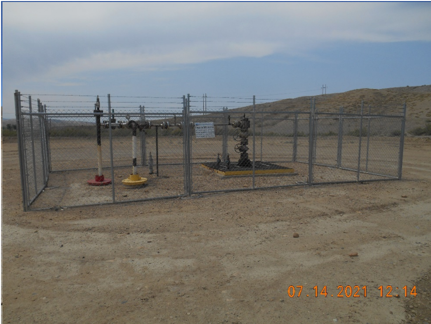
Injection wellhead.
