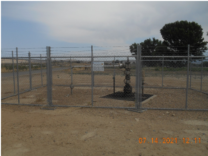
Injection wellhead
