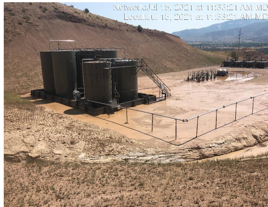
Photo #4440 Sediment encroaching on production equipment.
