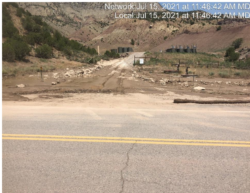
Photo #4455 No form of tracking BMP implemented.
