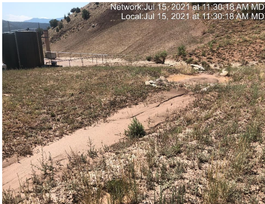
Photo #4437 Sediment trap filled with sediment.
