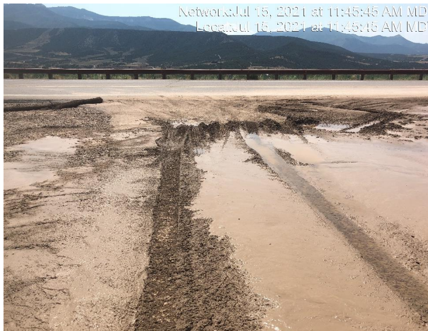
Photo #4454 No form of tracking BMP has been implemented.
