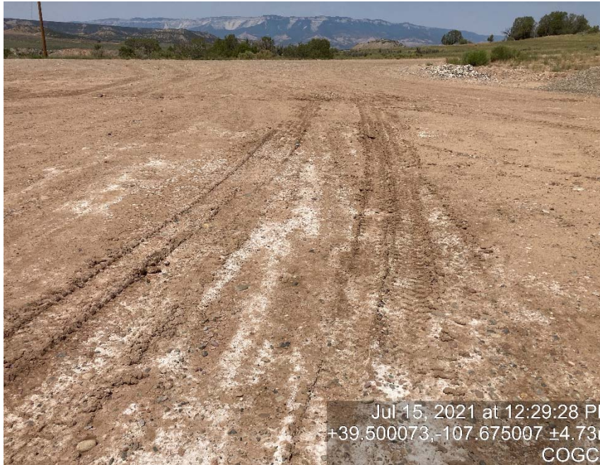
Lack of stabilization/compaction
