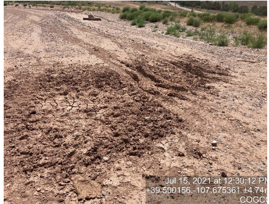
Lack of stabilization/compaction
