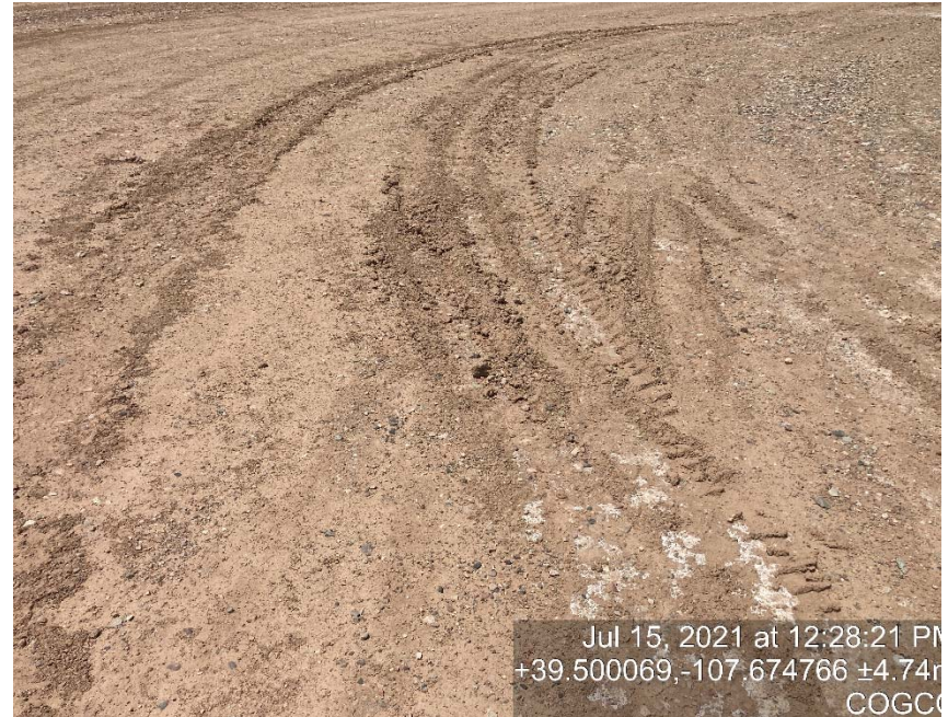
Lack of stabilization/compaction
