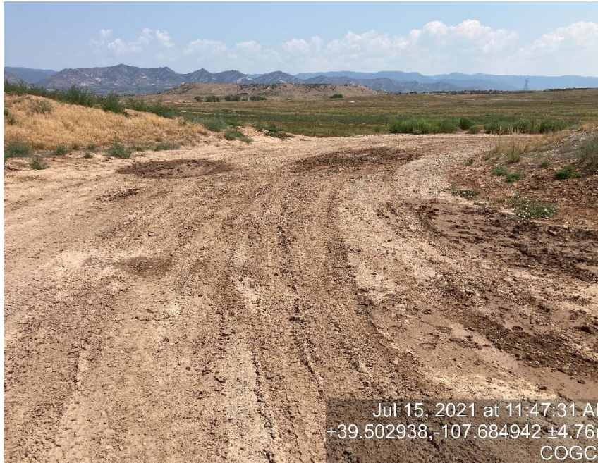
Lack of stabilization/compaction
