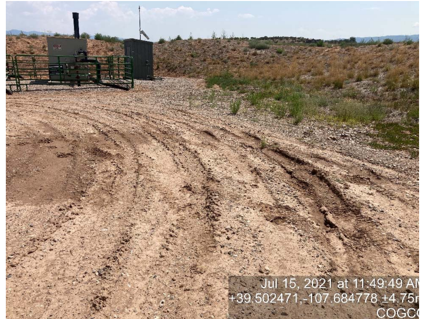
Lack of stabilization/compaction
