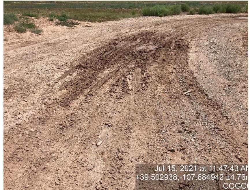
Lack of stabilization/compaction
