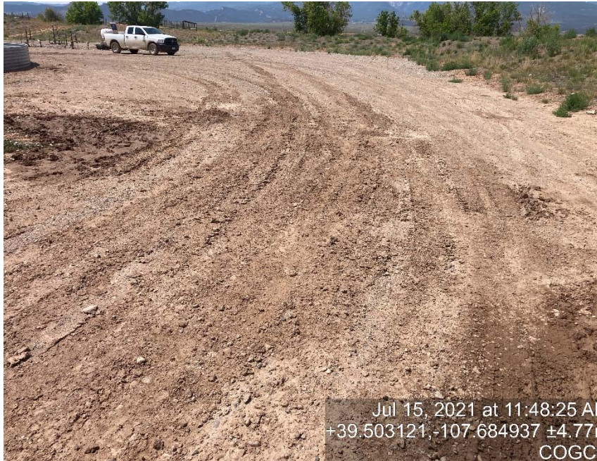
Lack of stabilization/compaction
