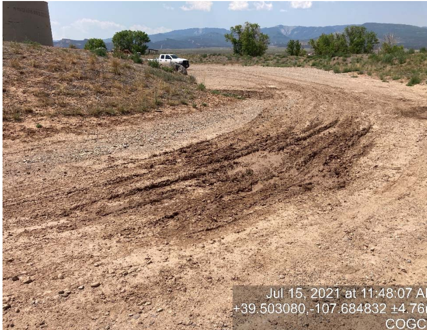
Lack of stabilization/compaction
