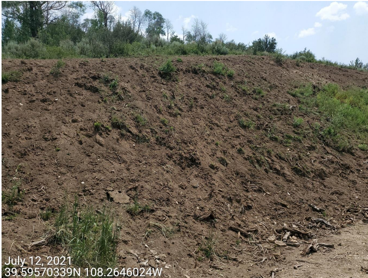
Photo 1: Photo taken from the cut slopes on the east end of the Location. Photo shows control measures to protect and stabilize slopes of the Location remain missing or insufficient; soils predominantly exposed and loose.
