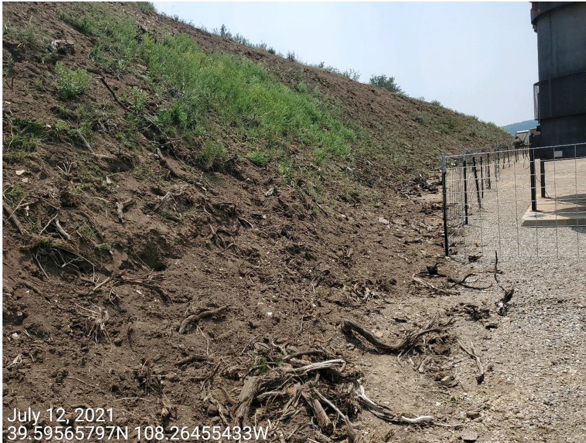
Photo 2: Photo taken from the cut slopes on the east end of the Location. Photo shows control measures to protect and stabilize slopes of the Location remain missing or insufficient; soils predominantly exposed and loose.
