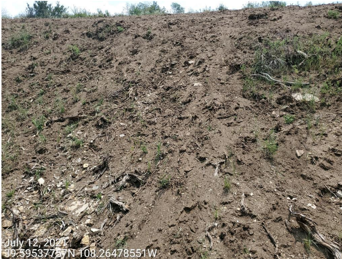
Photo 3: Photo taken from the cut slopes on the east end of the Location. Photo shows control measures to protect and stabilize slopes of the Location remain missing or insufficient; soils predominantly exposed and loose. Erosion degradation evident.
