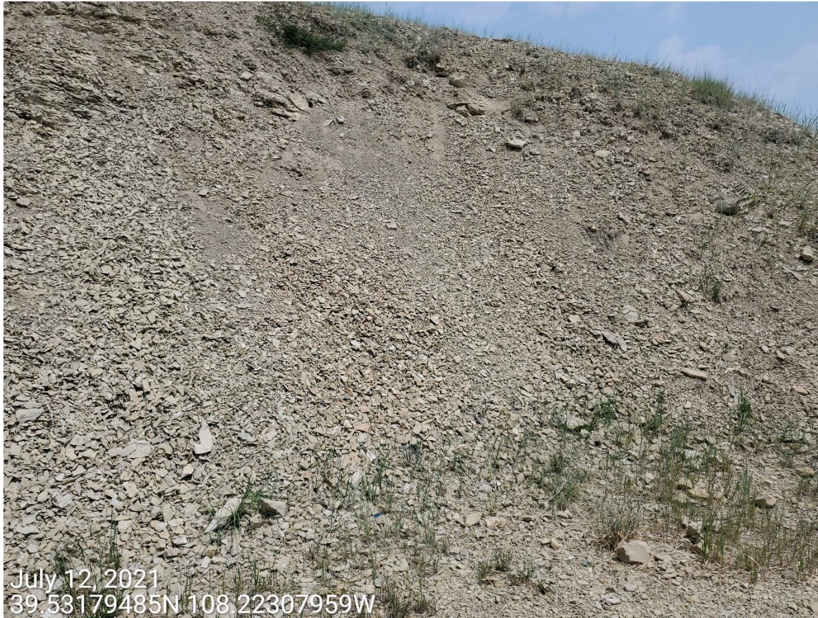
Photo 5: Photo taken from the cut slopes on the North end of the Location, facing north. Photo shows BMPs to protect and stabilize the cut slopes of the Location remain missing or insufficient.
