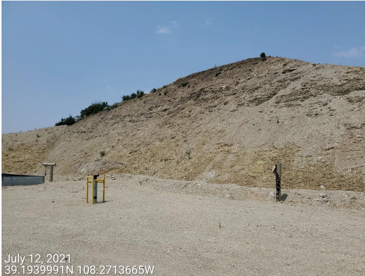
Photo 1: Photo taken from the Location, facing west. FIRR No. 402706390 shows Operator installed a soil binder and mulch on the cut slopes of the Location. Photo show BMP is not in proper functioning condition; BMP not adequate for the site's conditions to protect and stabilize cut slopes of the Location.
