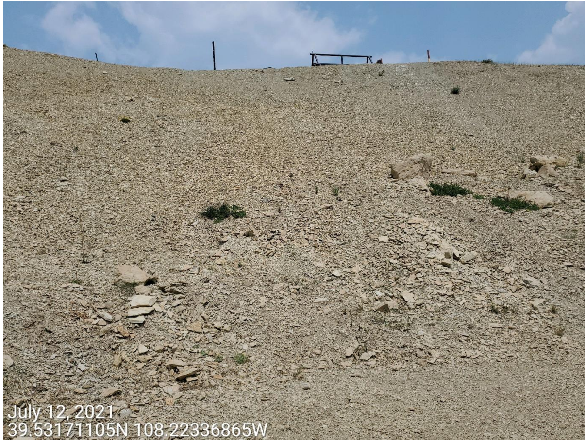
Photo 4: Photo taken from the cut slopes on the North end of the Location, facing north. Photo shows BMPs to protect and stabilize the cut slopes of the Location remain missing or insufficient.
