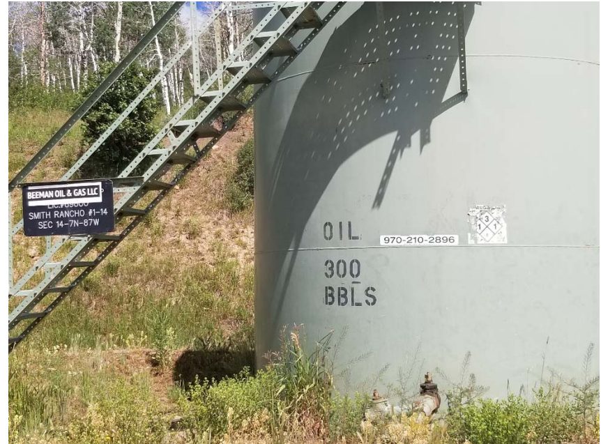
Photo 4. Battery sign not updated to current sign rule. Tank label not updated to current tank label rule.
