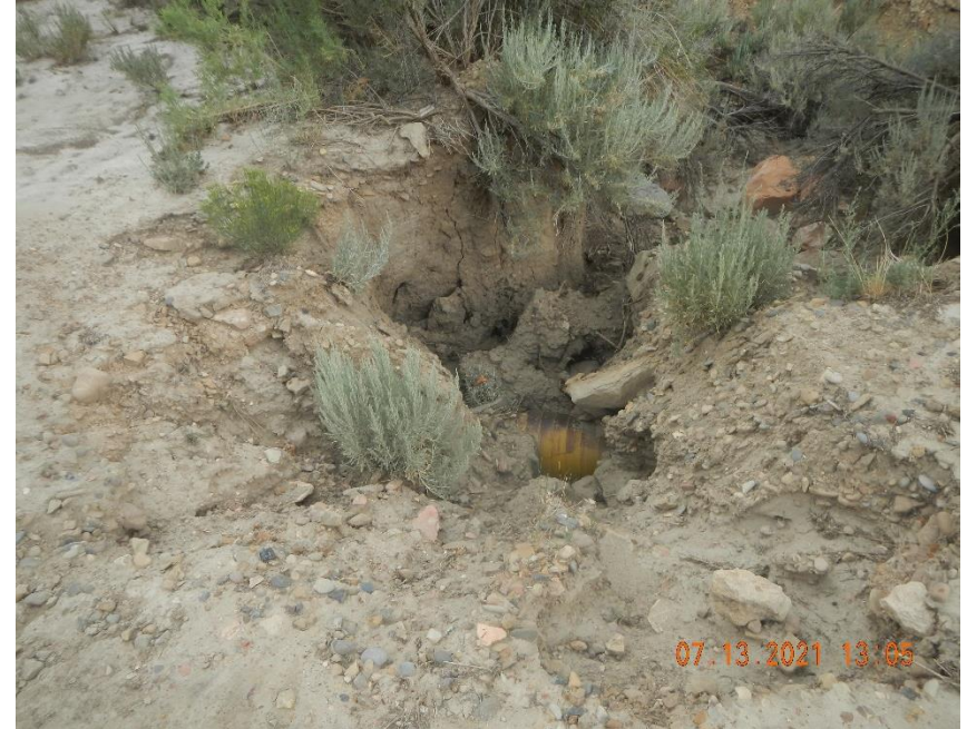
Shoulder of road is washing away and exposing gas line. 39.83447 108.80650
