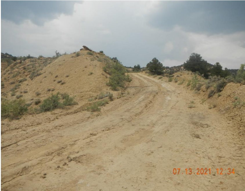
Erosion of road at the entrance of location.
