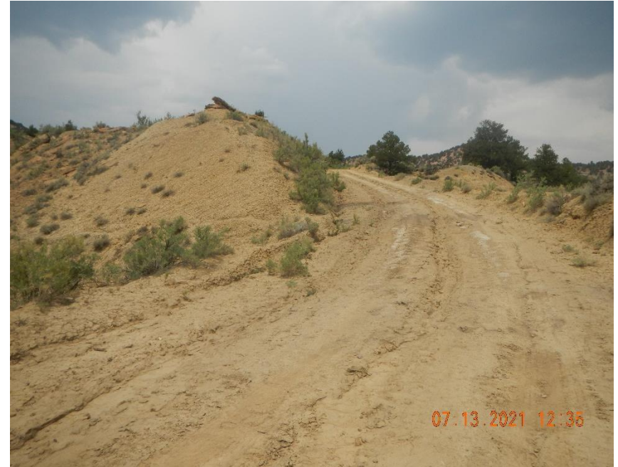
Access roads and BMPs not maintained in a stable condition.
