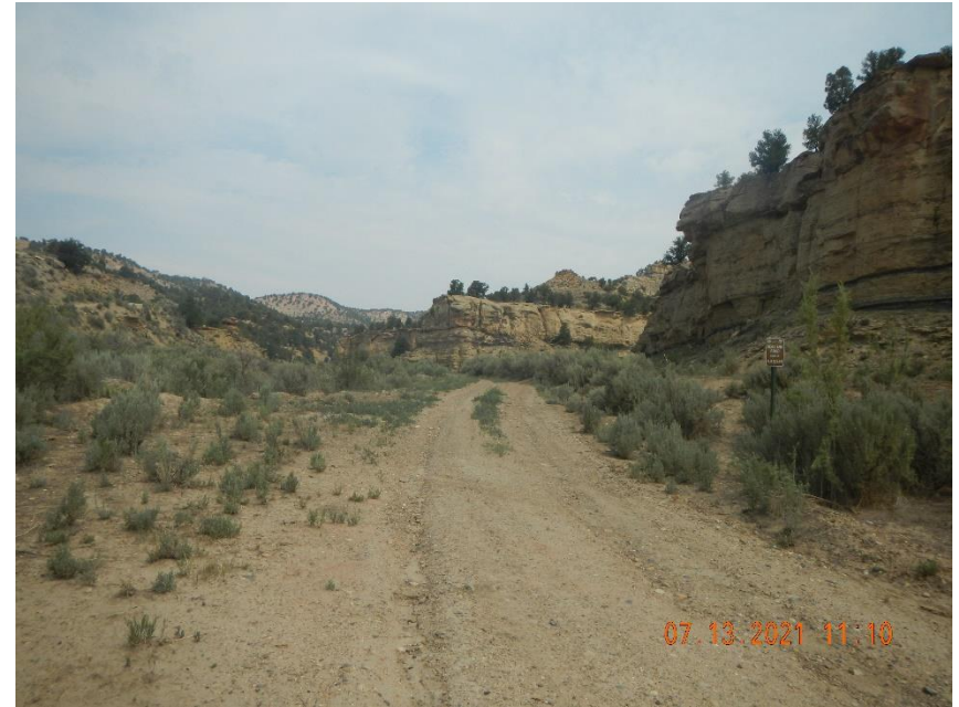
Erosion of road and movement of sediment.
