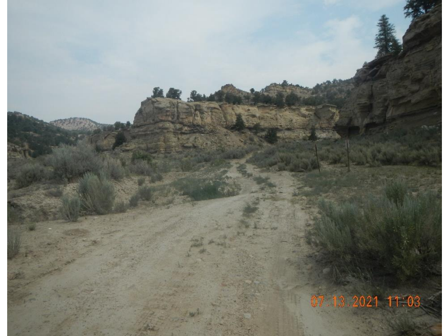
Movement of sediment on access road.
