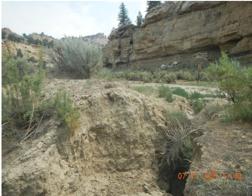
Wash out from erosion rill crossing access road.
