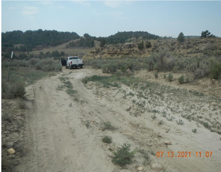
Erosion rill crossing access road. Weeds on access road.
