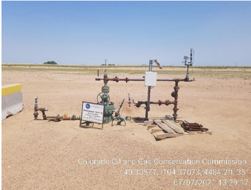
Photo 7 – Middlepark 18-21-3L Wellhead
