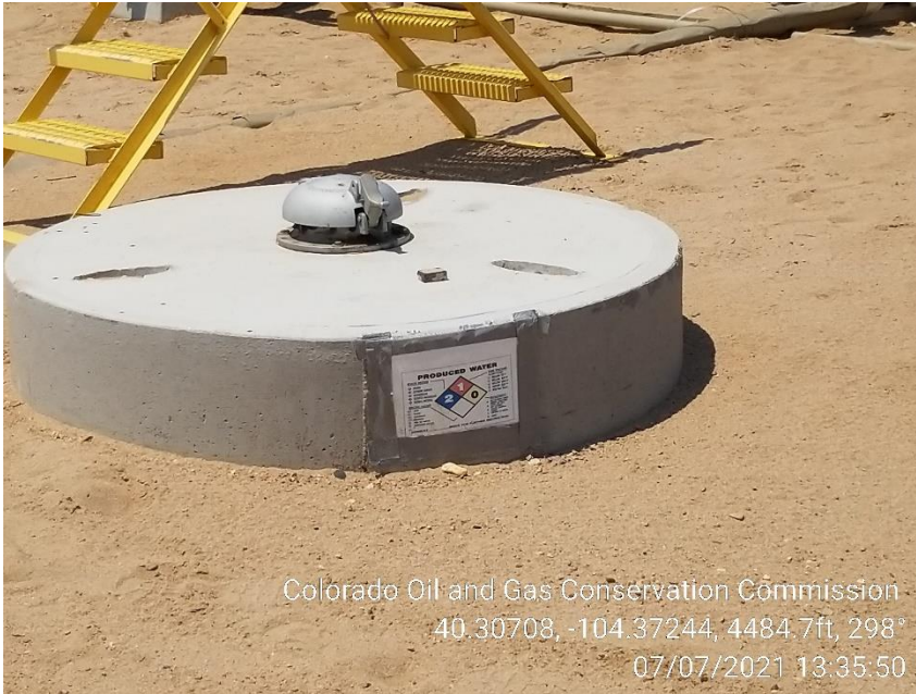
Photo 17 – Compressor Drain Pit missing Capacity Label
