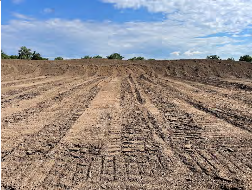
Photograph: 1 | Facing North
