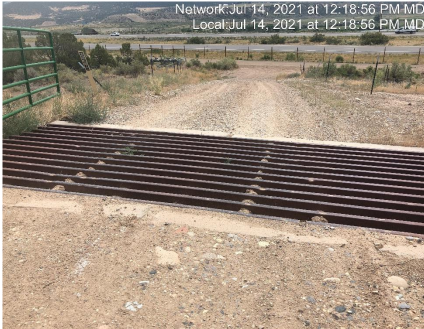
Photo #4423 Tracking BMP insufficient.
