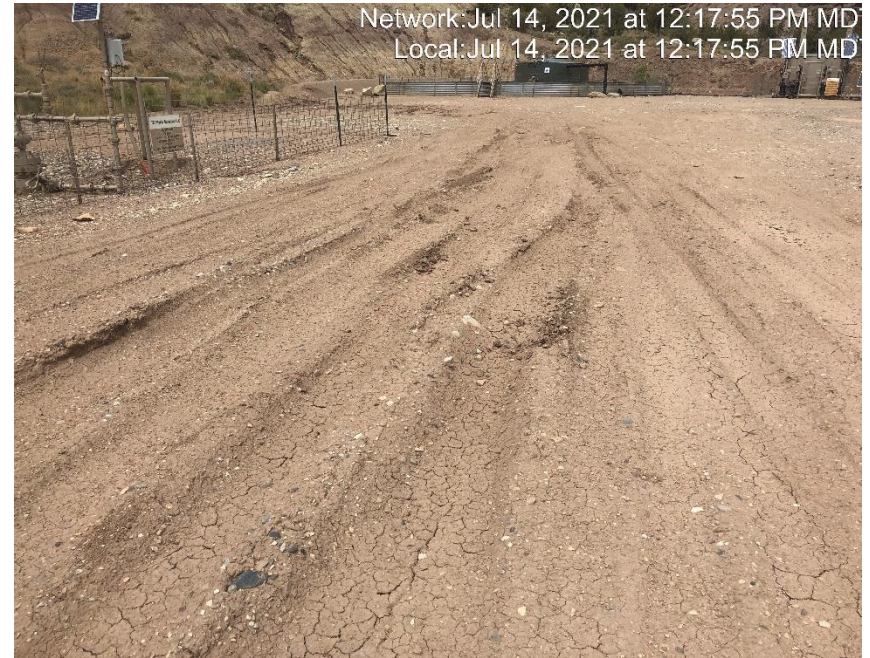
Photo #4421 Location lacks stabilization.
