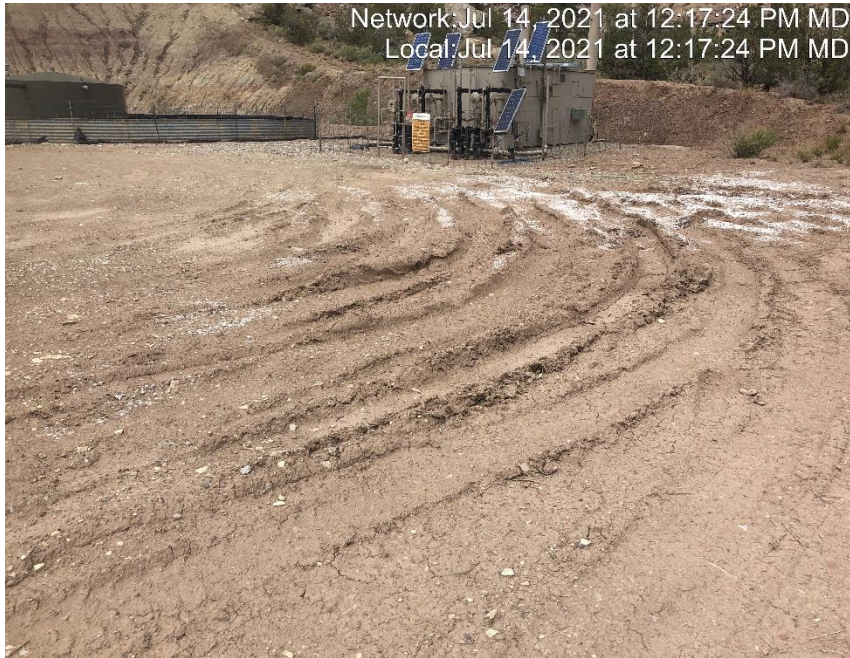
Photo #4420 Location lacks stabilization.
