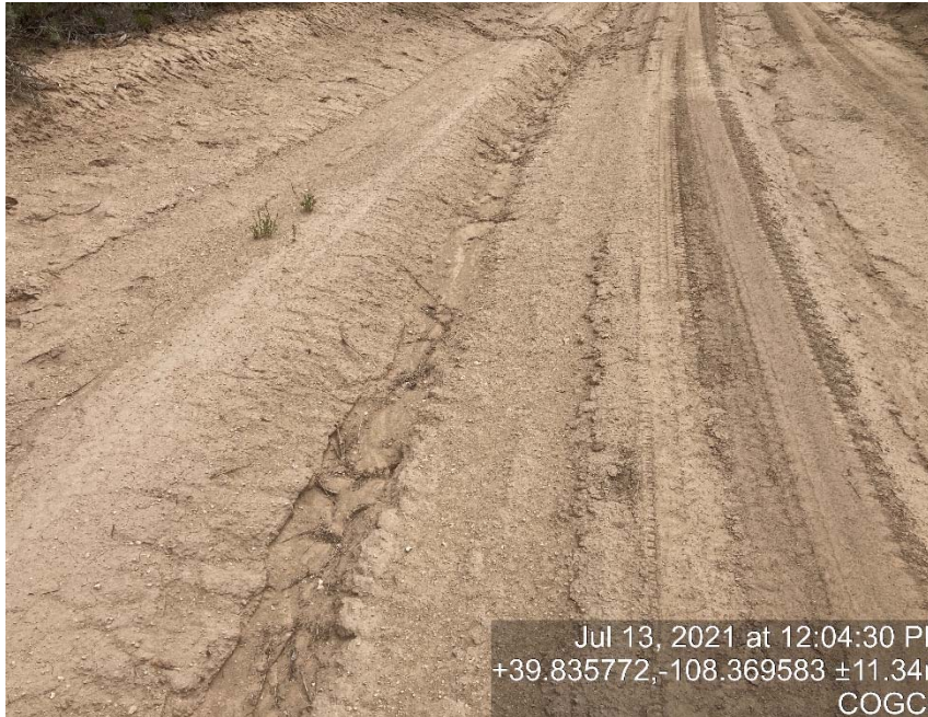
Access road lack of stabilization/compaction and erosion
