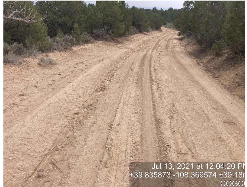
Access road lack of stabilization/compaction and erosion
