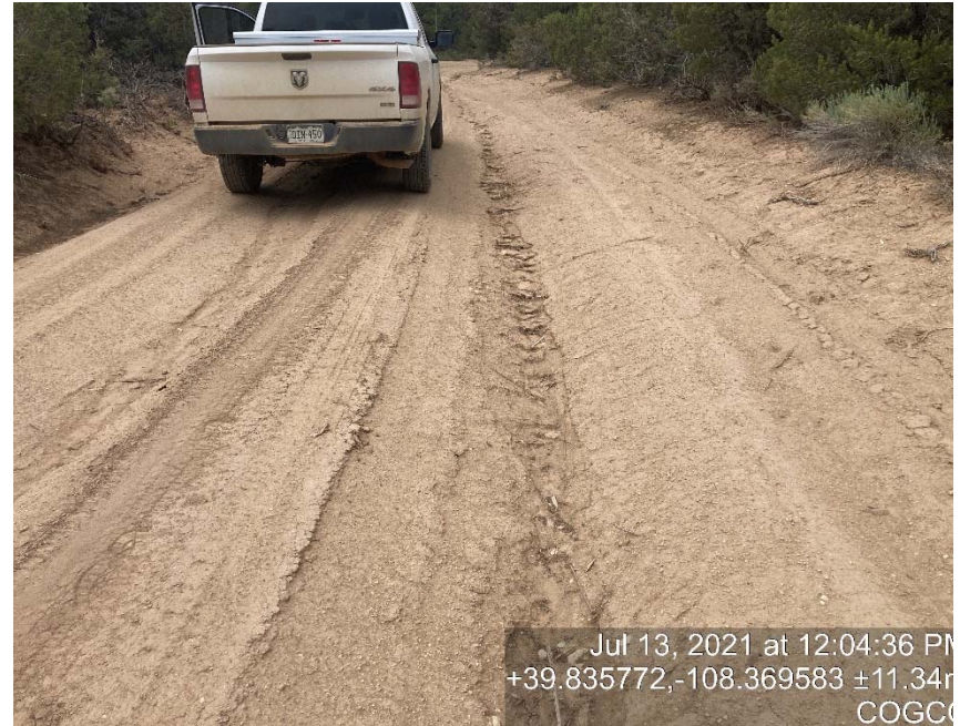
Access road lack of stabilization/compaction and erosion
