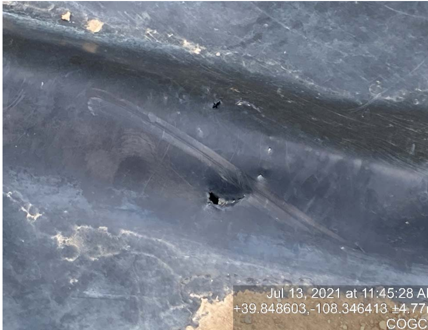
Hole in tank containment on base
