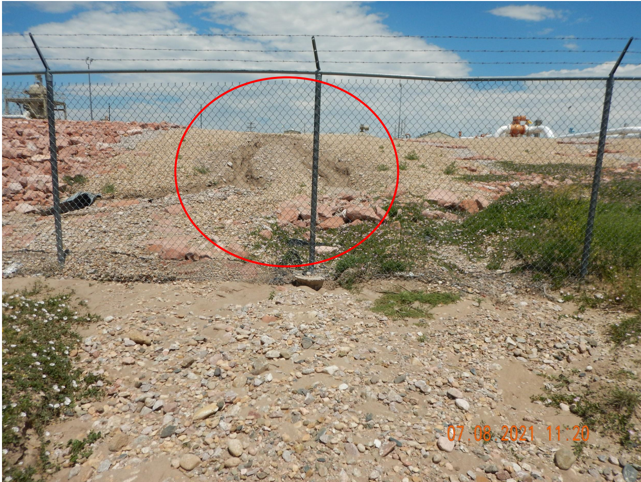
Photo 4. Photo taken from the southern Cheyenne Compressor Station, facing North. Photo illustrates unmanaged stormwater erosion coming off the location going around some adjacent rip-rap.
