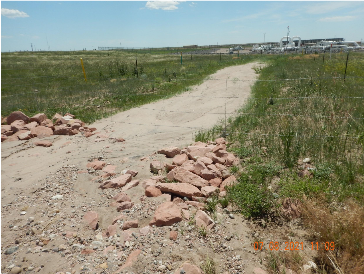
Photo 10. Photo taken from the southern reach of the stormwater erosion, facing South. Photo illustrates impacts to recent stormwater and reclamation work that has been impacted by unmanaged stormwater runoff from the Cheyenne Compressor Station.
