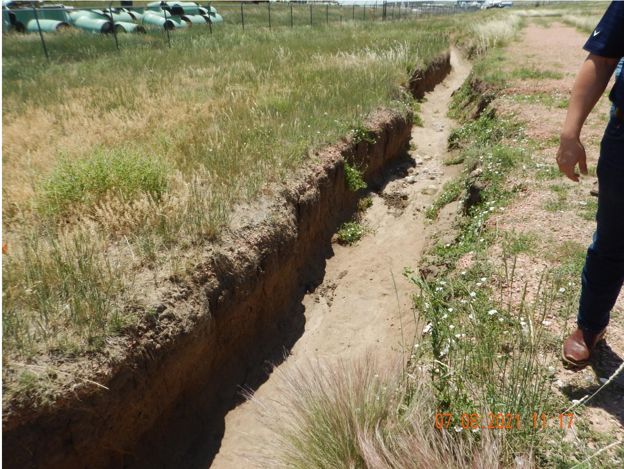
Photo 8. Photo taken from the southern property boundary of the Cheyenne Compressor Station, facing South. Photo illustrates the stormwater erosion impacts coming off the location and causing gully erosion and impacting the downgradient surface owners. This portion of the reach is a safety hazard for cattle operations and exposed buried lines from the adjacent facilities.
