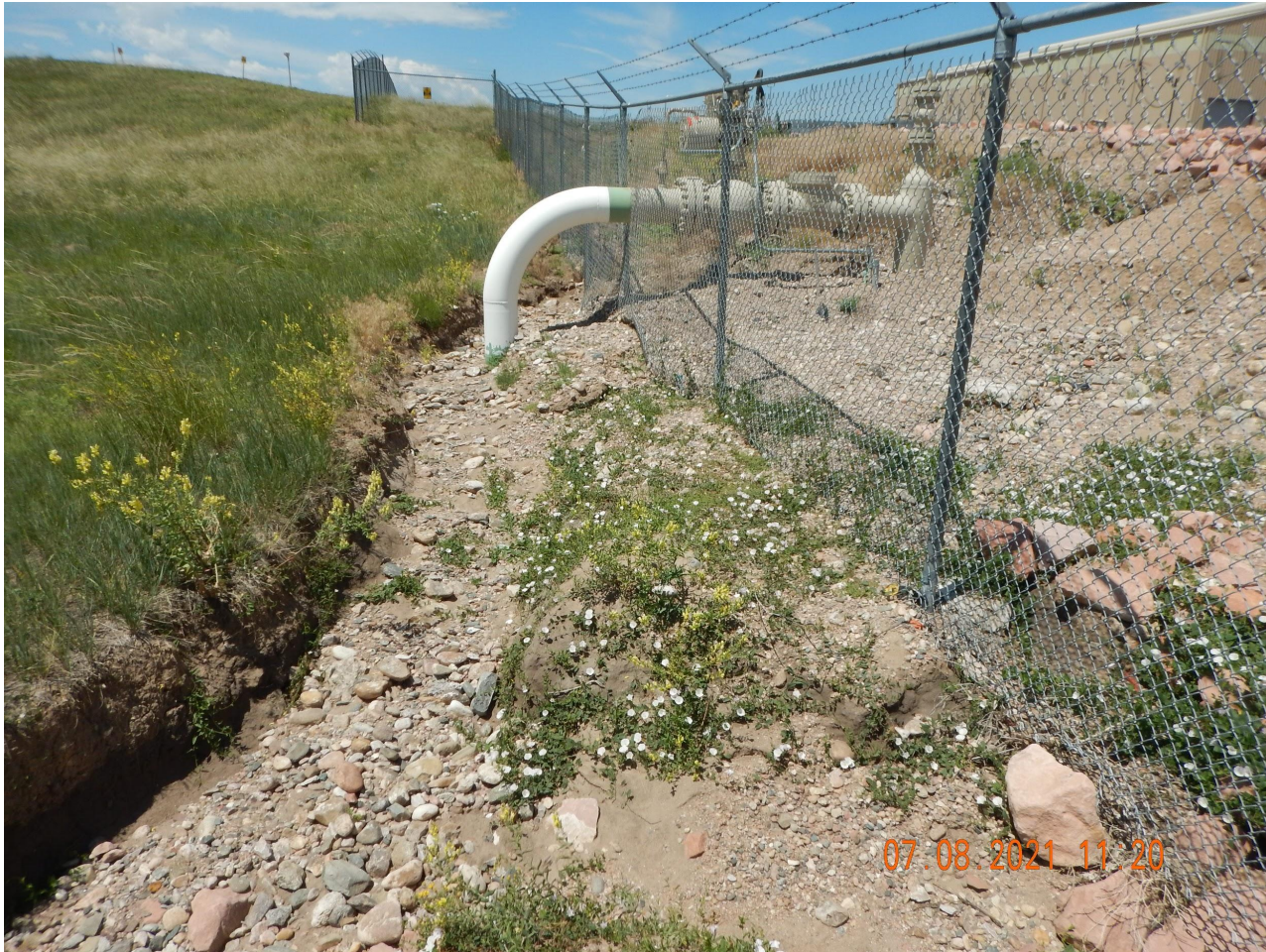
Photo 5. Photo taken from the southern Cheyenne Compressor Station, facing West. Photo illustrates unmanaged stormwater erosion coming off the location and causing gully erosion.
