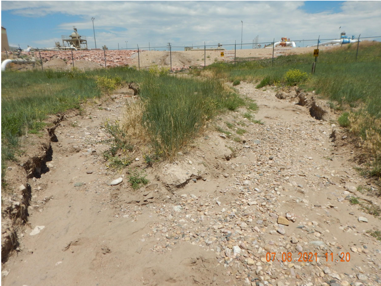
Photo 6. Photo taken south of the Cheyenne Compressor Station, facing North. Photo illustrates the stormwater erosion impacts coming off the location and causing gully erosion.
