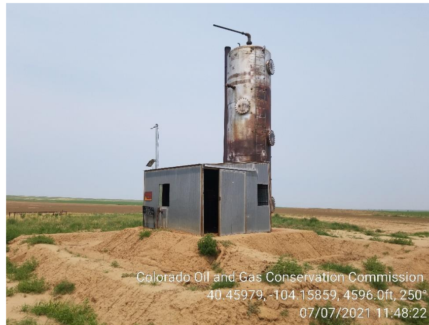
Photo 6 – Heater Treater – Berms installed
