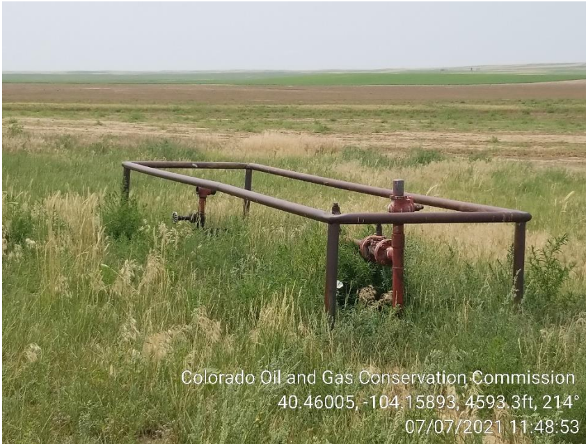
Photo 7 – Manifold – Weed Re-Growth – Unused Pipe has been removed
