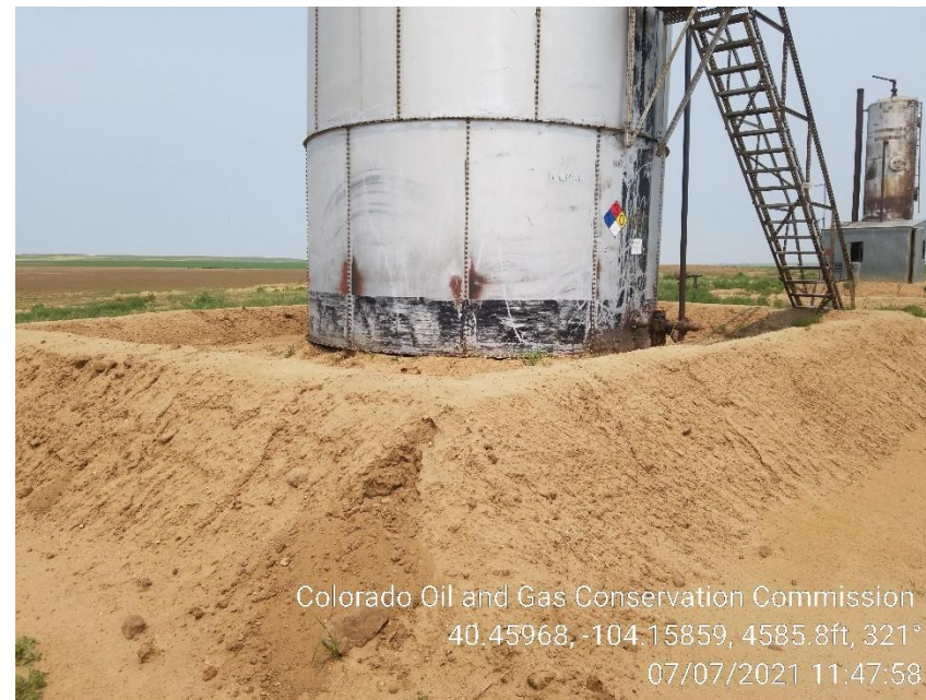
Photo 4 – Berms Repaired
