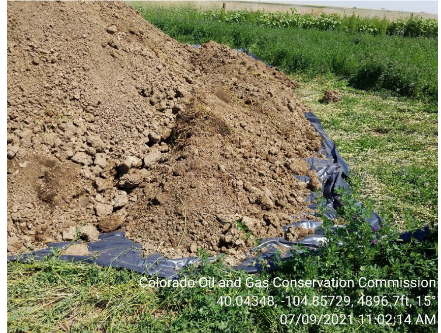
Photo 8 – Impacted soil being placed on plastic liner then transported off-site.
