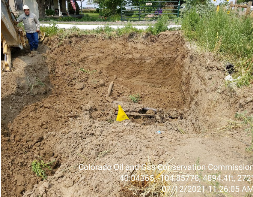
Photo 7 - Spill excavation 7/12; soil impacts remain in-situ.
