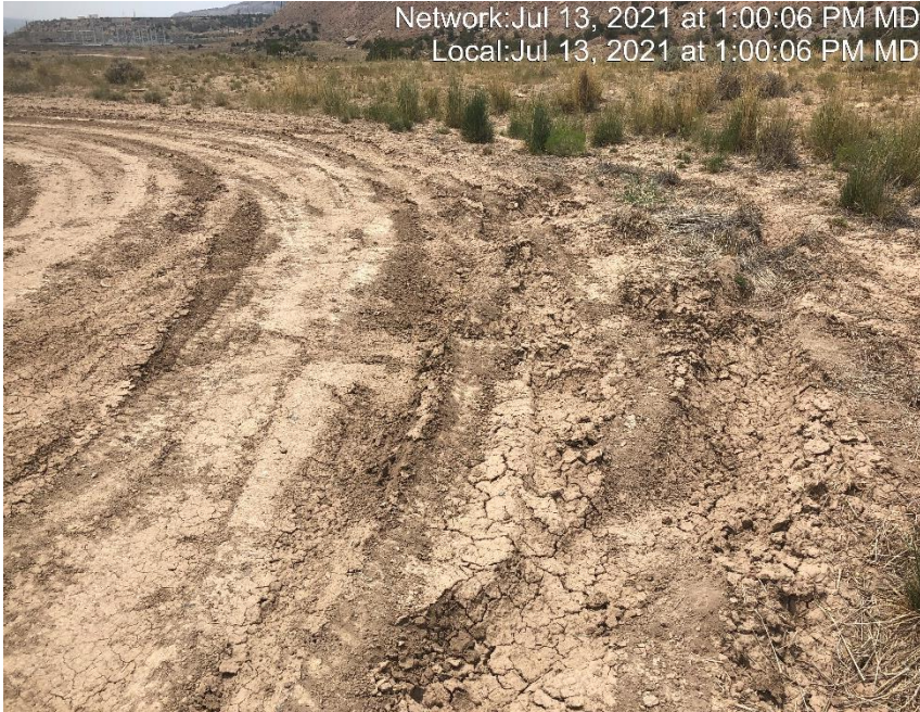
Photo #4411 Location lacks stabilization.
