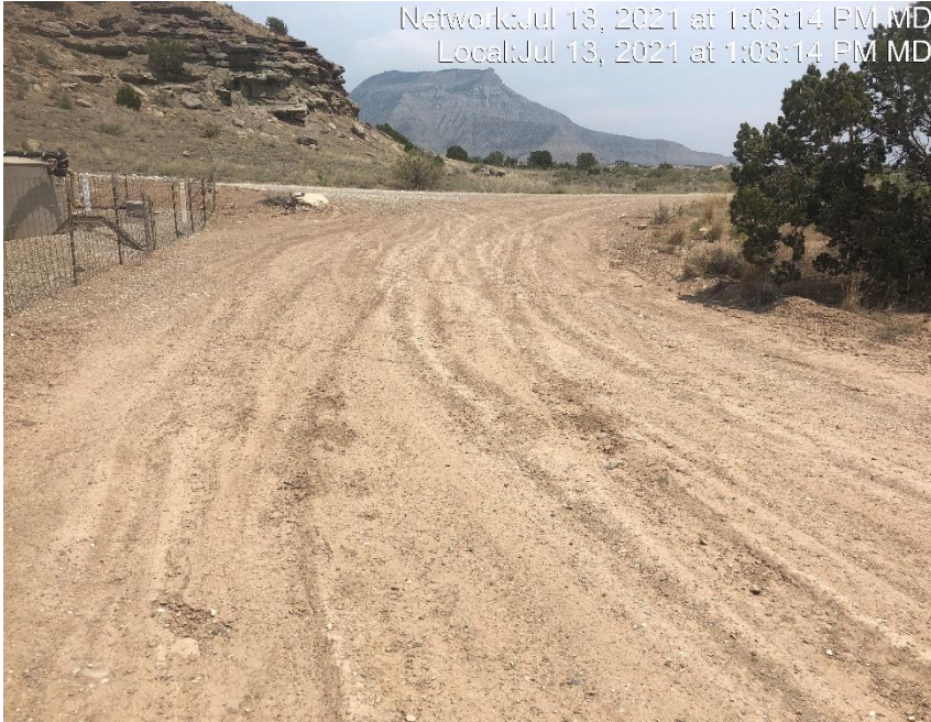
Photo #4413 No form of tracking BMP located at entrance to location.
