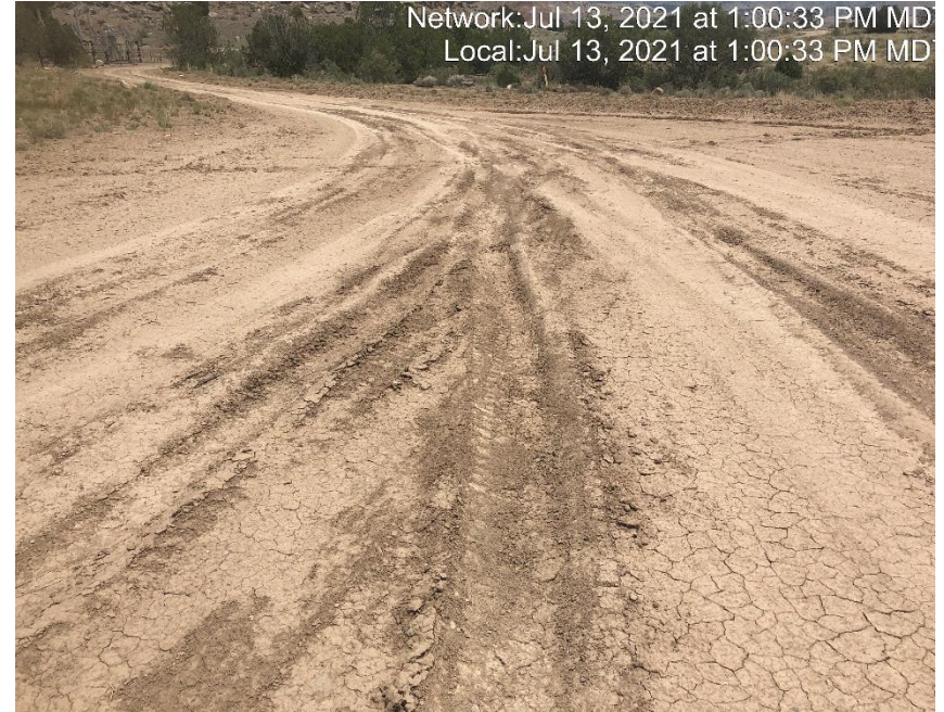
Photo #4412 Location lacks stabilization.
