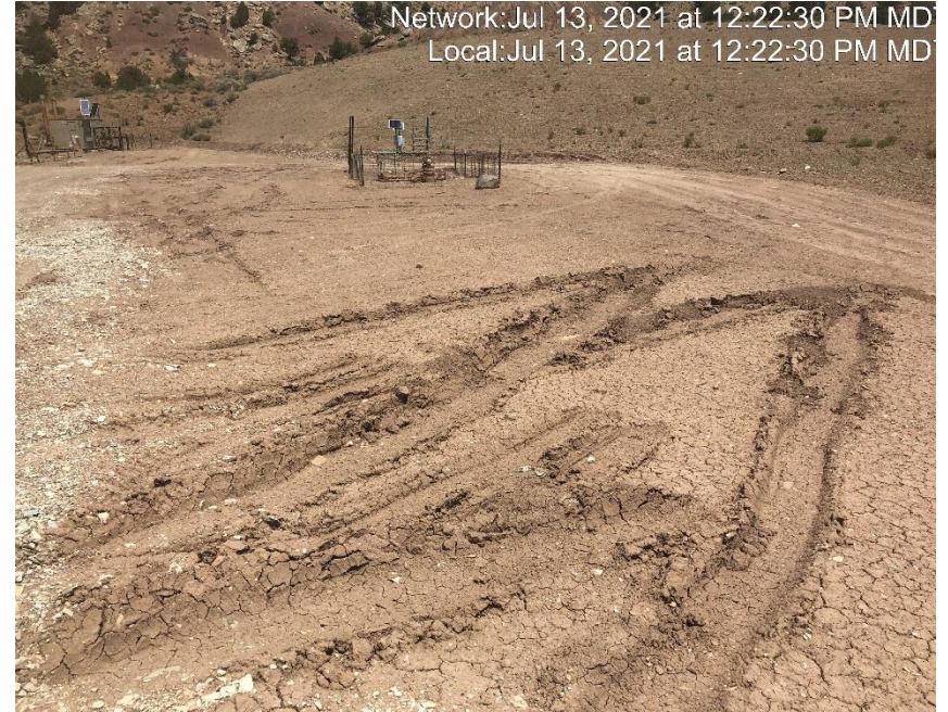
Photo #4407 Location lacks stabilization.
