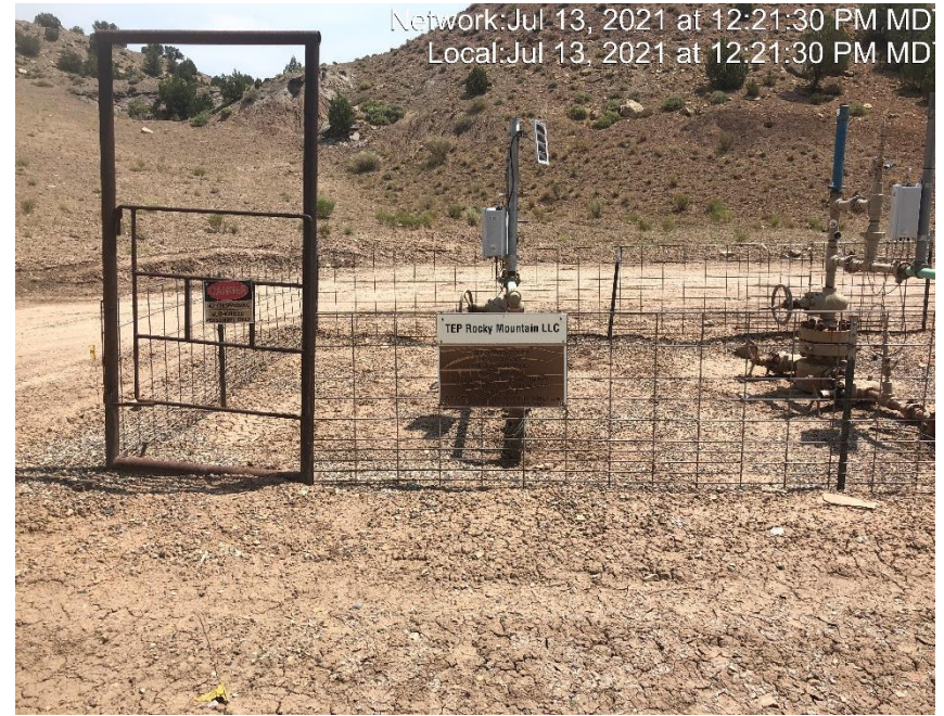
Photo #4405 Well head sign weathered and not legible.
