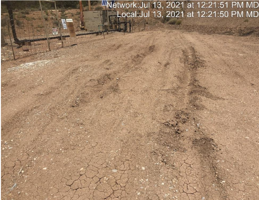
Photo #4406 Location lacks stabilization.
