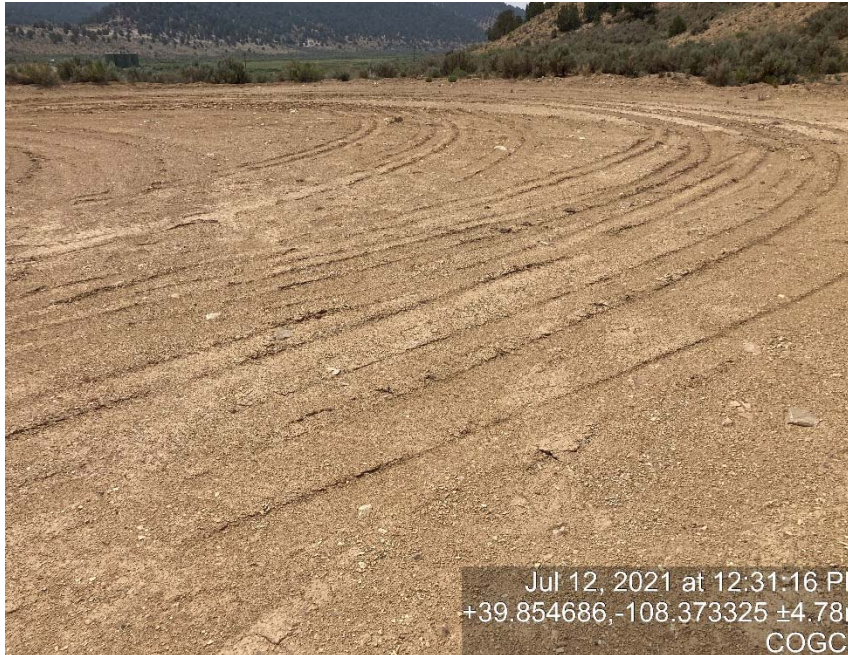
Lack of stabilization/compaction
