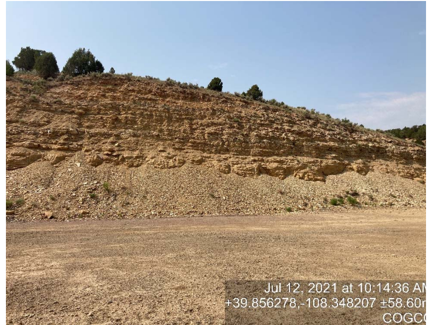
Lack of stabilization on cut slope
