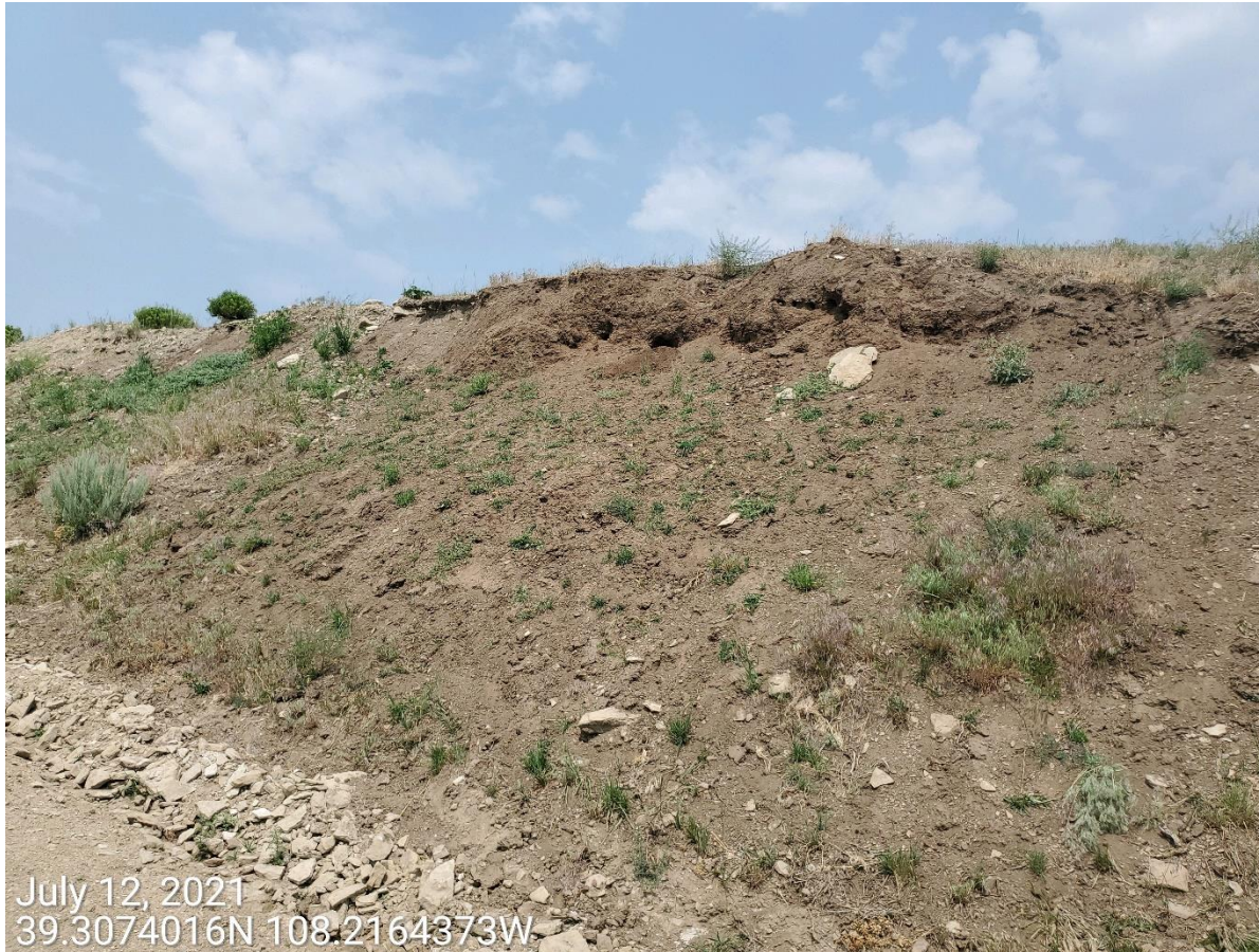
Photo 7: Photo taken from the fill slopes of the Location. Photo shows control measures to protect/stabilize slopes of the Location are missing or insufficient.
