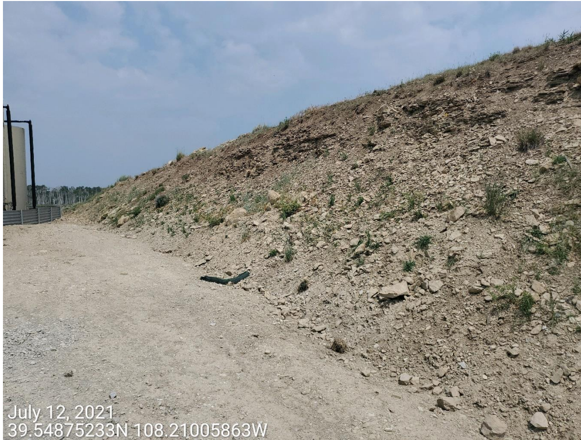
Photo 8: Photo taken from the cut slopes on the east end of the Location. Photo shows control measures to protect/stabilize slopes of the Location are missing or insufficient.
