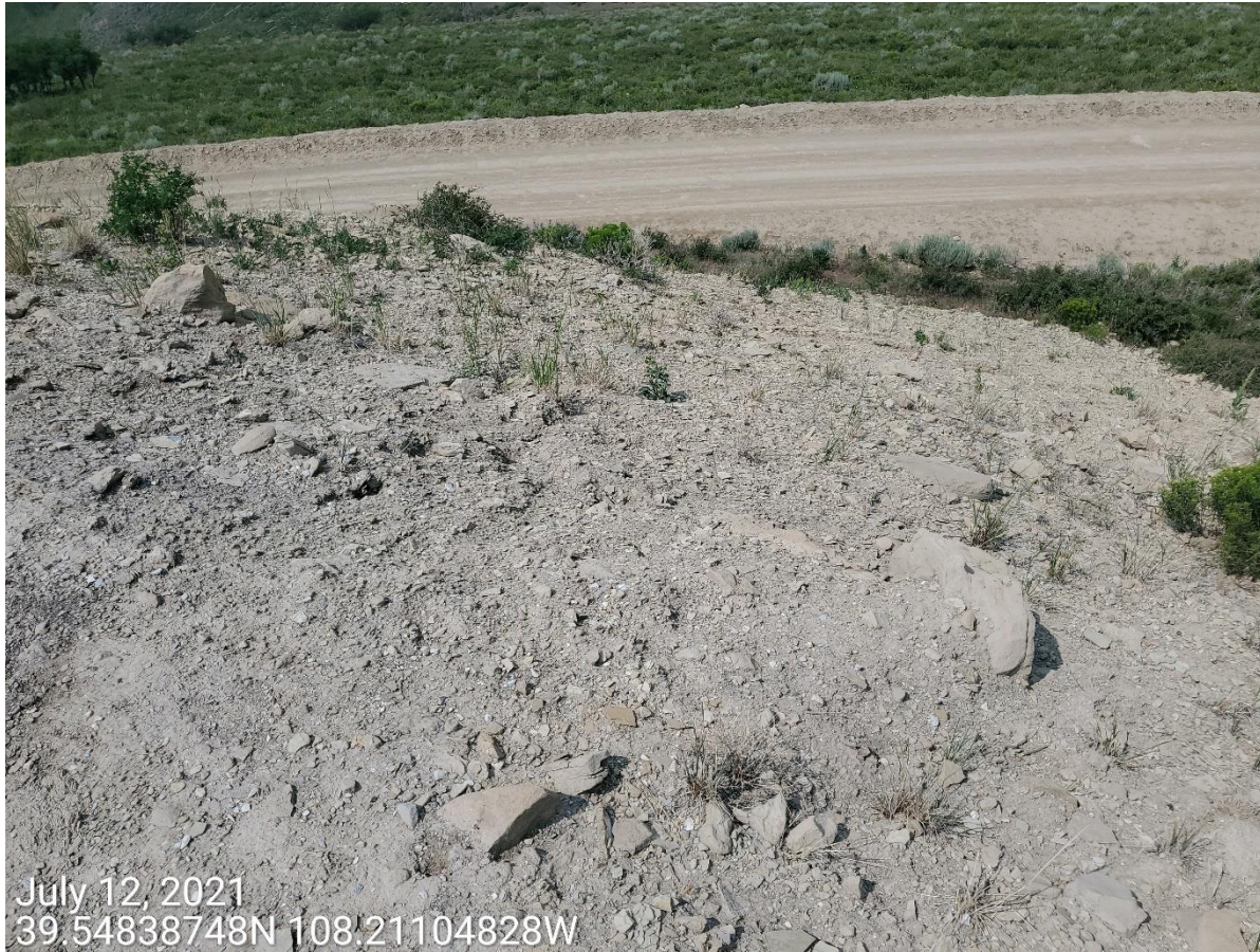
Photo 6: Photo taken from the fill slopes of the Location. Photo shows control measures to protect/stabilize slopes of the Location are missing or insufficient.
