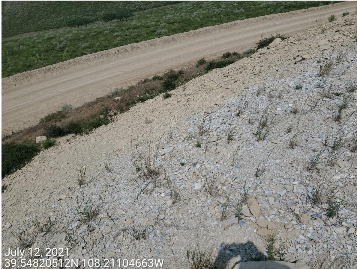
Photo 5: Photo taken from the fill slopes of the Location. Photo shows control measures to protect/stabilize slopes of the Location are missing or insufficient.
