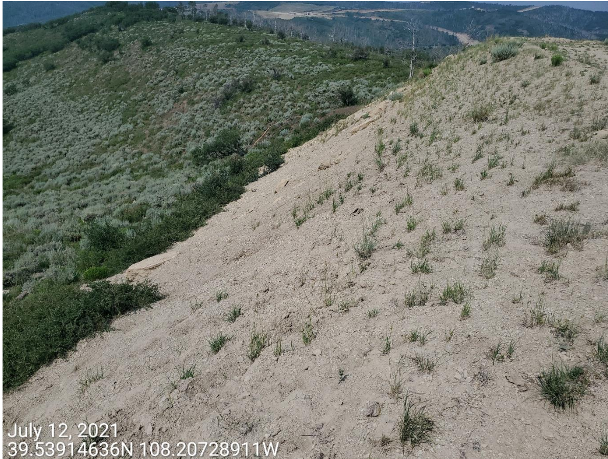
Photo 5: Photo taken from the south end of the Location, facing west. Photo shows control measures to protect/stabilize the fill slopes of the Location remain missing or insufficient.
