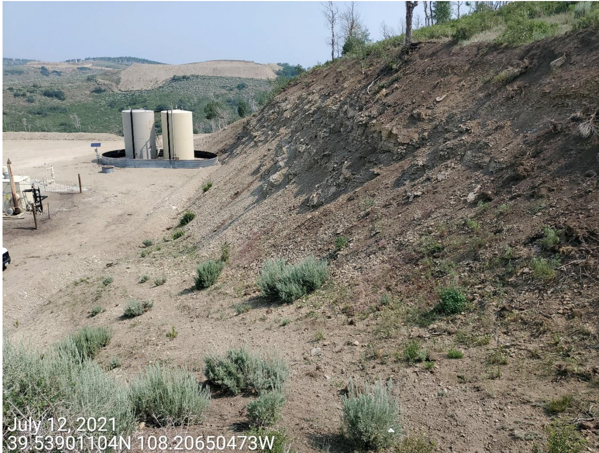
Photo 3: Photo taken from the east end of the Location, facing north. Photo shows control measures to protect/stabilize the cut slopes of the Location remain missing or insufficient.
