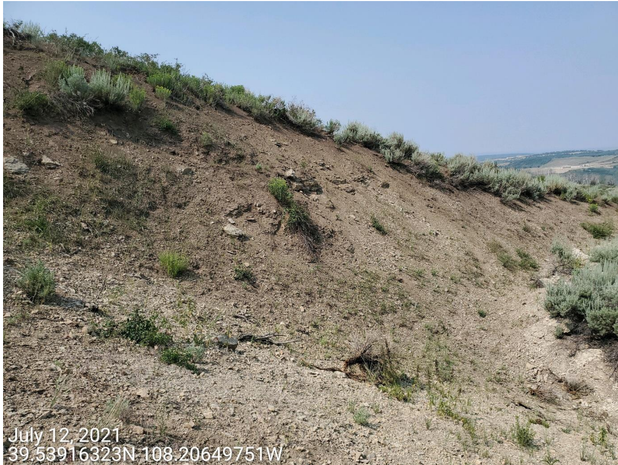
Photo 4: Photo taken from the east end of the Location, facing southwest. Photo shows control measures to protect/stabilize the cut slopes of the Location remain missing or insufficient.
