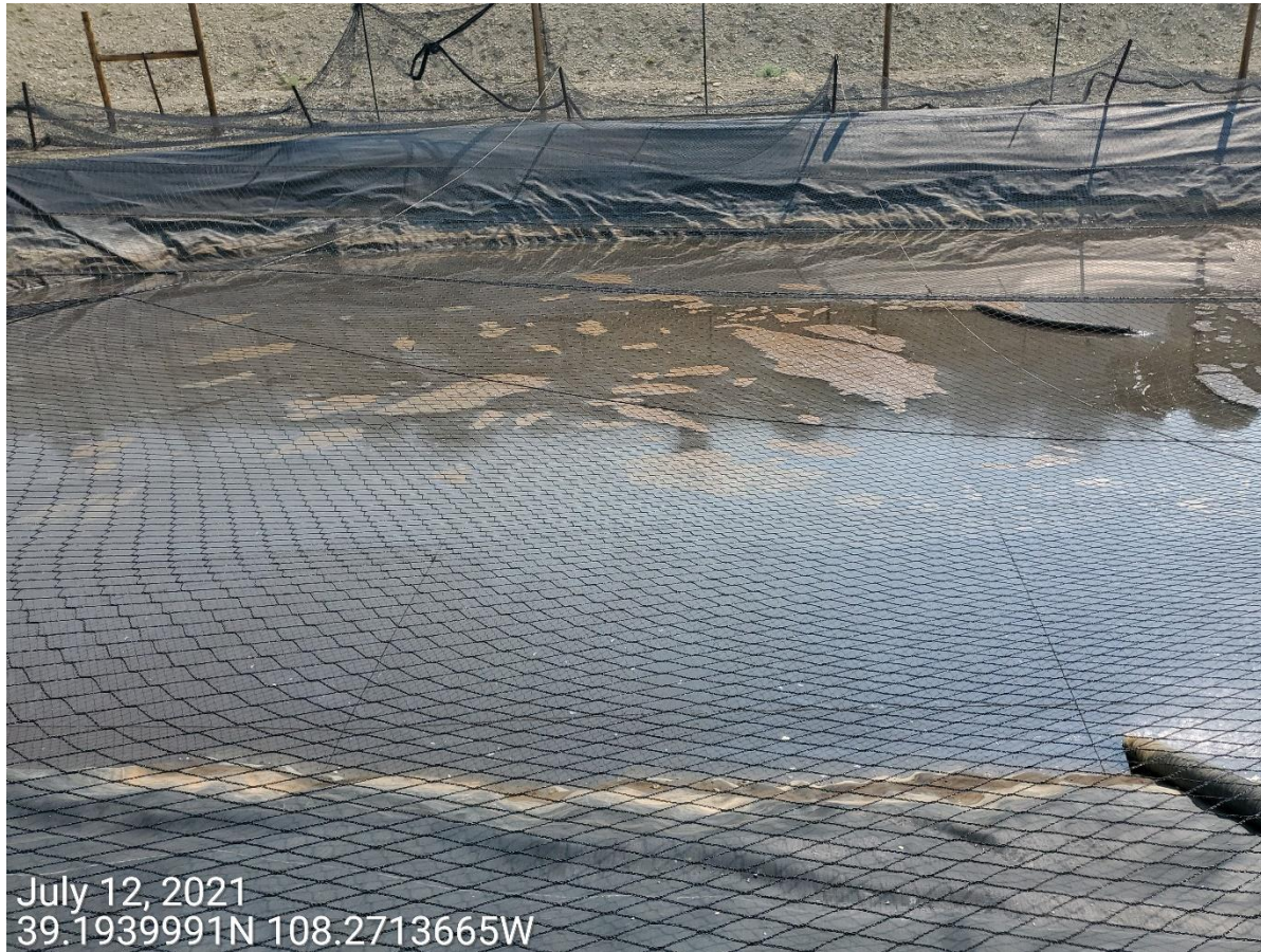
Photo 13: Photo shows hydrocarbon accumulation within the pit on Location.
