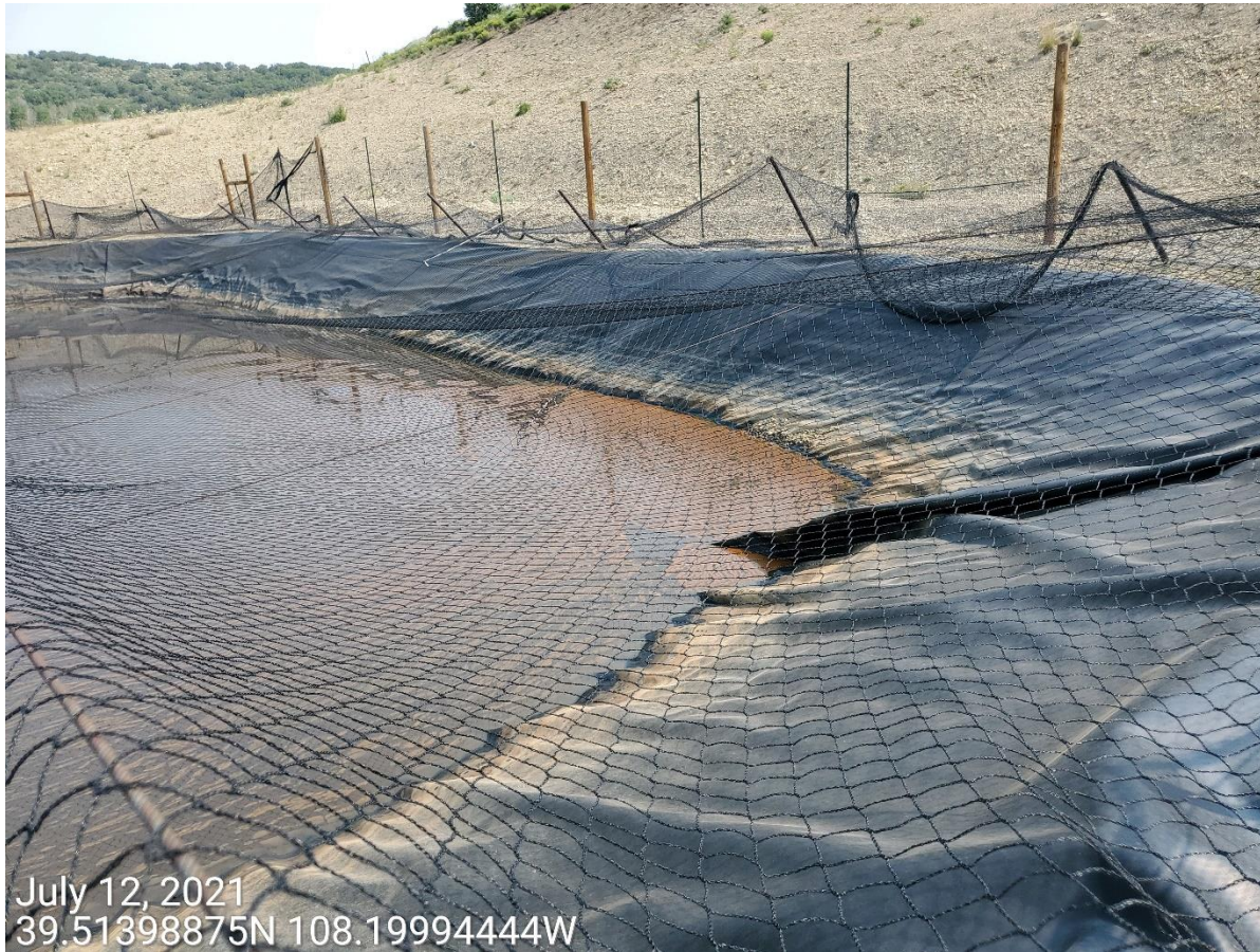
Photo 14: Photo shows hydrocarbon accumulation within the pit on Location.
