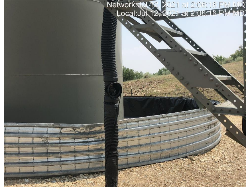
Photo #4399 heating insulation open ended and not capped.
