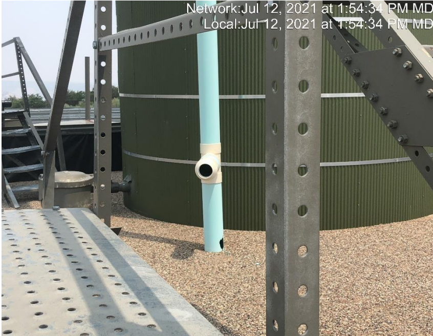
Photo #4392 Flow line heating insulation open ended and not capped.
