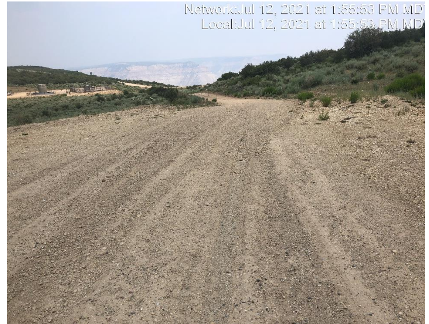
Photo #4395 No form of tracking BMP located at the entrance to location.
