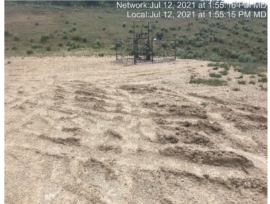
Photo #4393 Location lacks stabilization.
