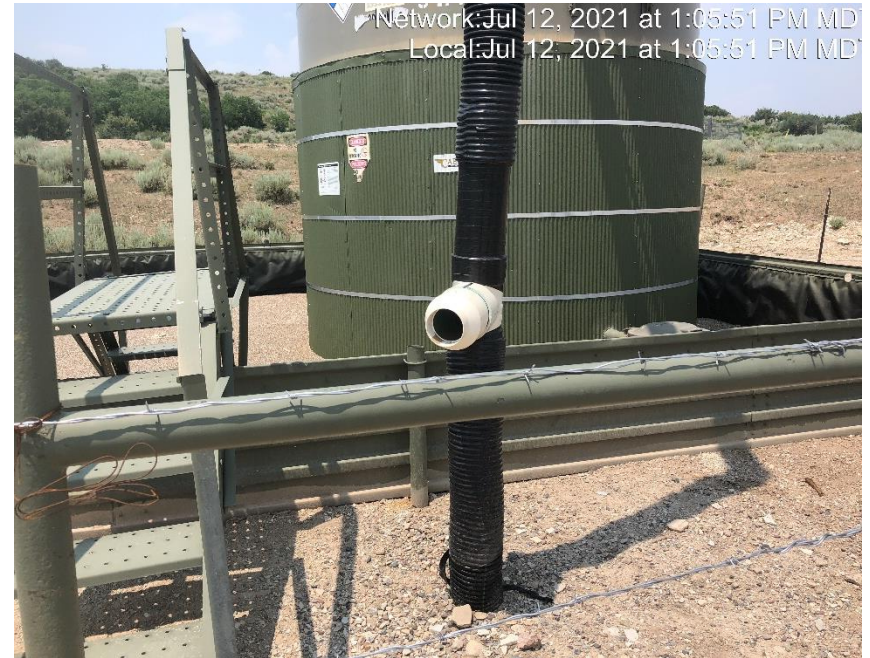
Photo #4386 flow line heating insulation opened ended and not capped.
