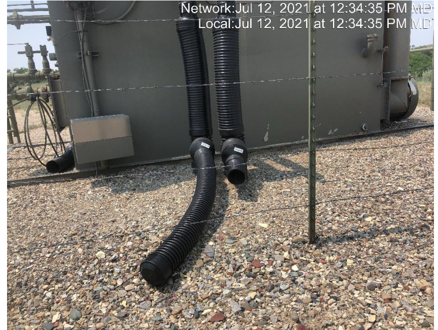
Photo #4383 Flow line heating insulation open ended and not capped.
