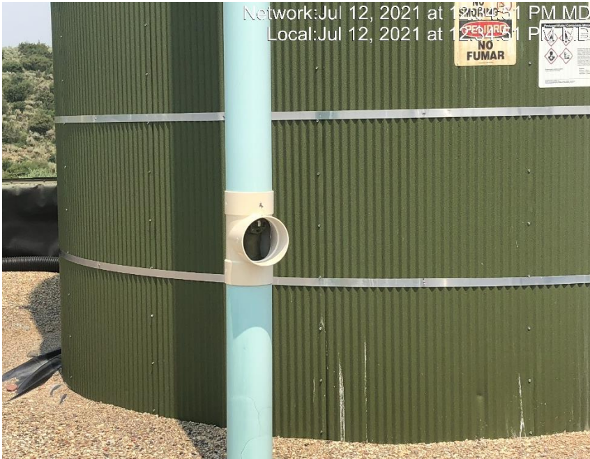
Photo #4384 Flow line heating insulation open ended and not capped.
