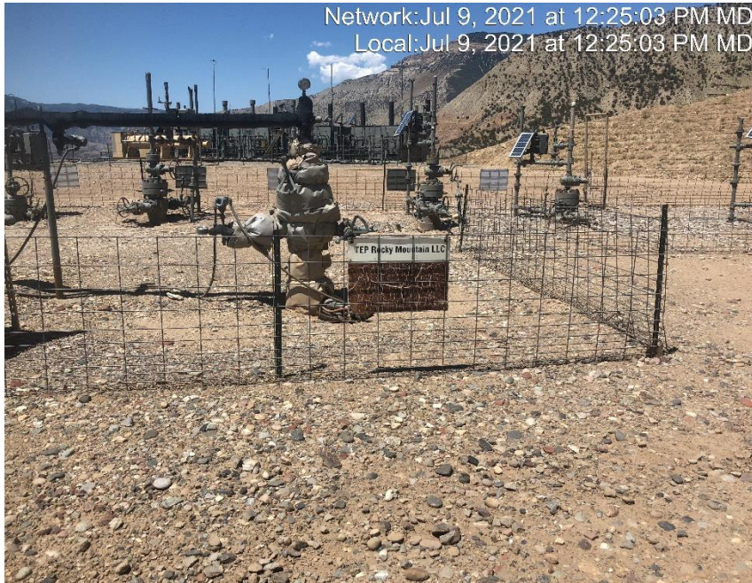
Photo #4376 Wellhead sign weathered and not legible.
